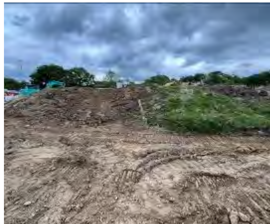
Photo 4 SP1 taken looking east
