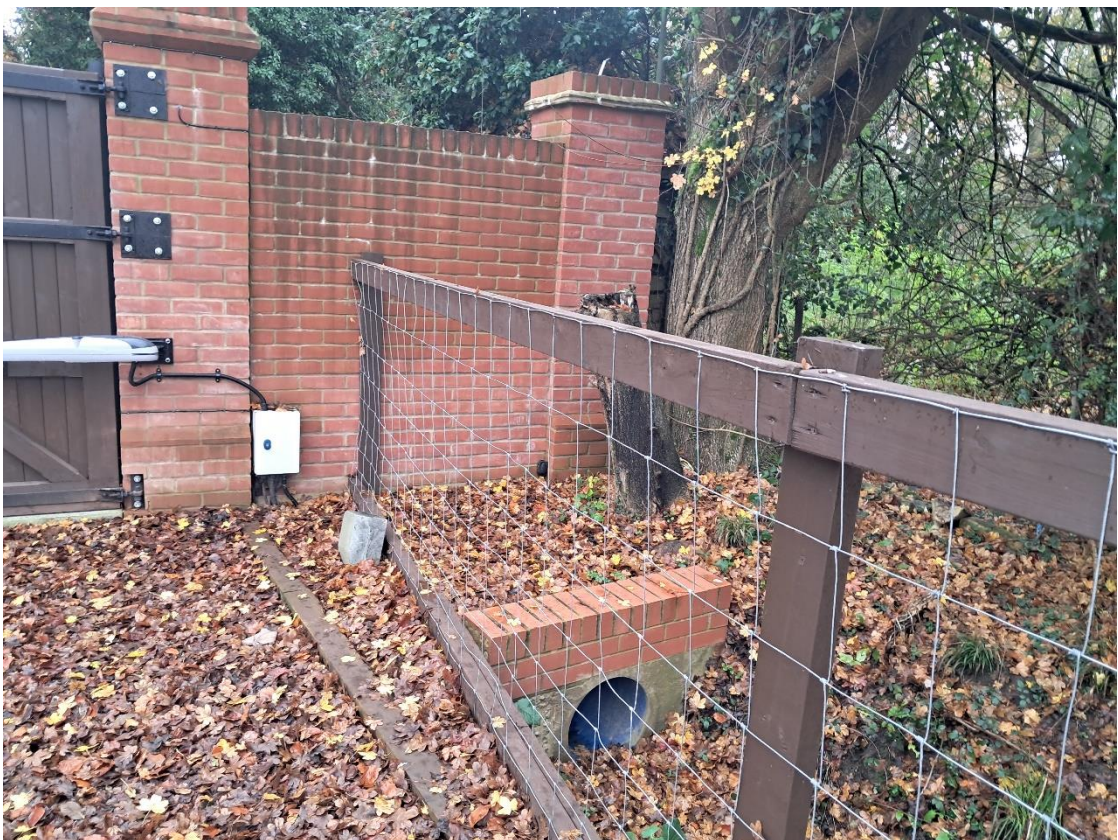
Photo 2 – Proximity of T044 (Field Maple) to new wall and replacement Culvert
