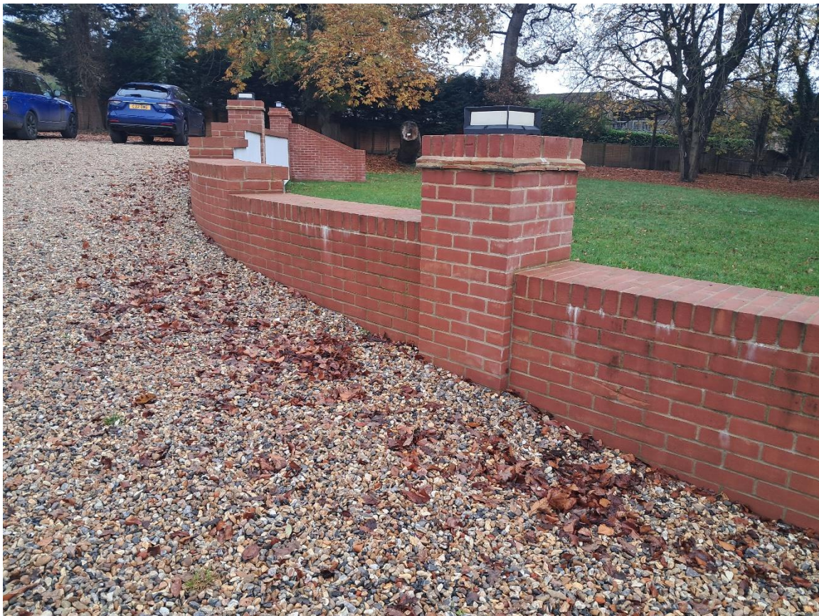
Photo 5 – Replacement retaining wall to the front of Woodlands Farm House.
