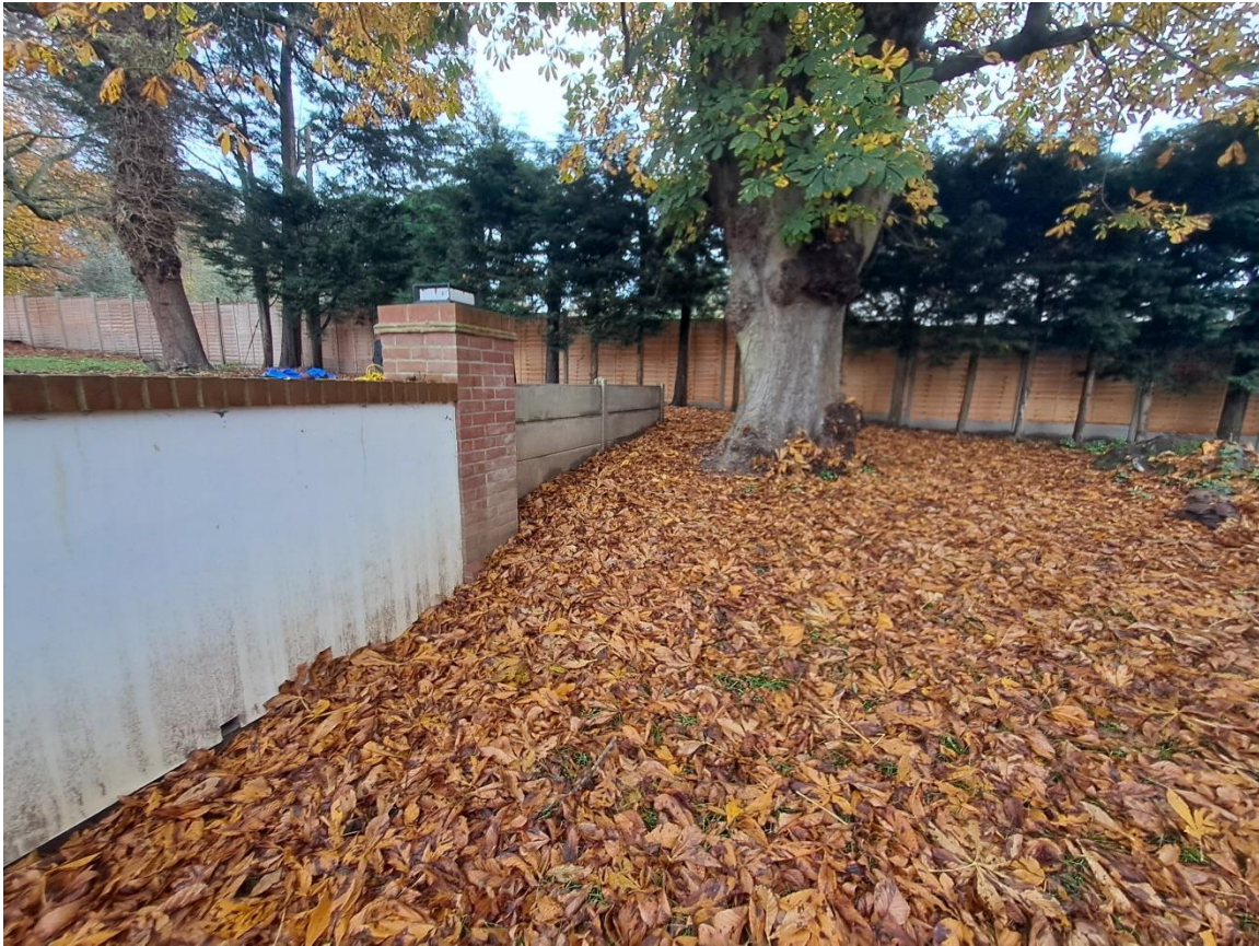
Photo 4 – Replacement retaining wall to the front of Woodlands Farm House.
