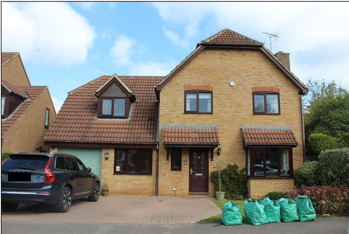
Photograph 1 – Front elevation as viewed from Payley Drive
