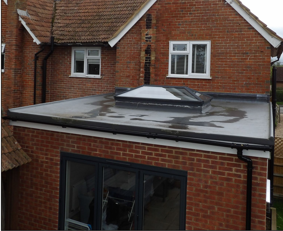
Figure 10. Sealed uPVC fascias on rear extension. 2 Diddenham Cottages, Grazeley. 01.10.24
