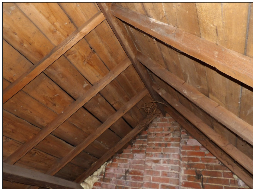
Figure 12. Example of timber sarking in loft space. 2 Diddenham Cottages, Grazeley. 01.10.24
