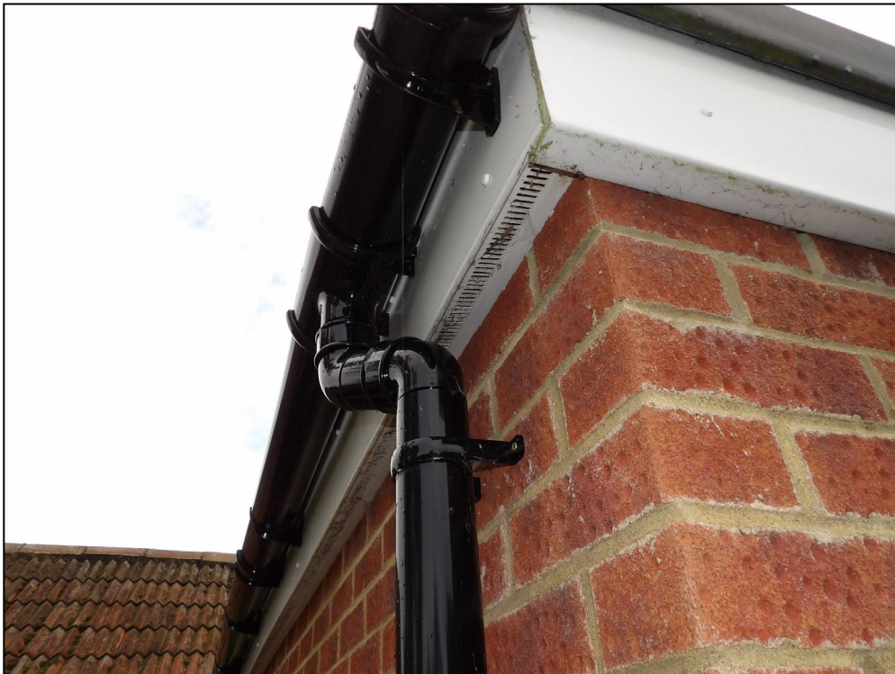
Figure 10. Sealed uPVC fascias on rear extension. 2 Diddenham Cottages, Grazeley. 01.10.24
