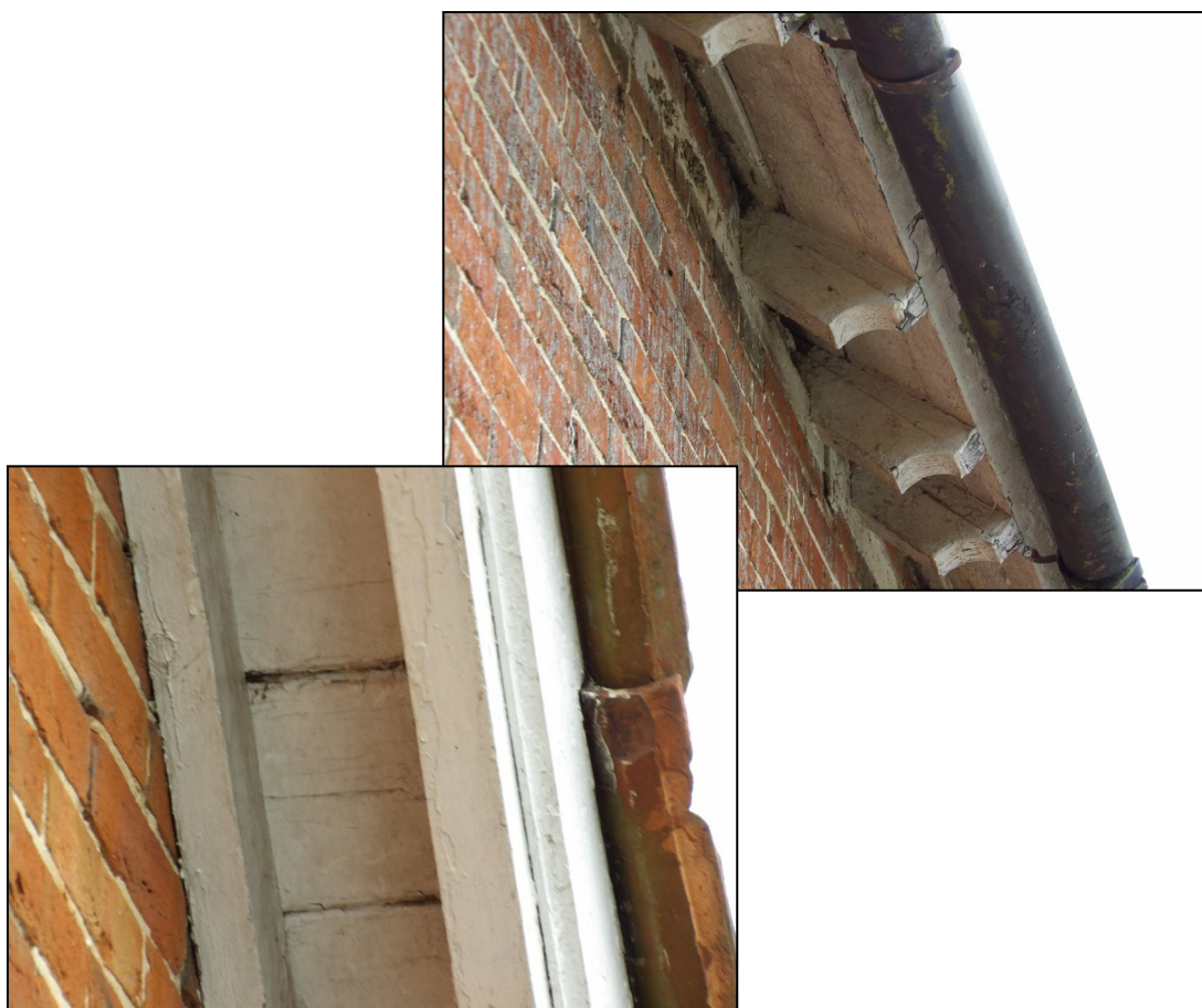
Figure 8. Example sealed eaves. 2 Diddenham Cottages, Grazeley. 01.10.24
