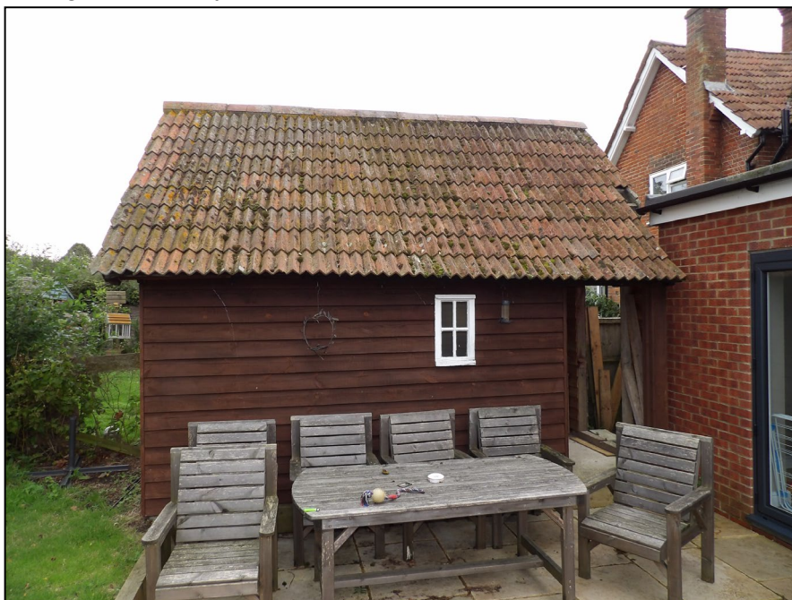
Figure 3. Rear single storey building not being affected by the works. 2 Diddenham Cottages, Grazeley. 01.10.24
