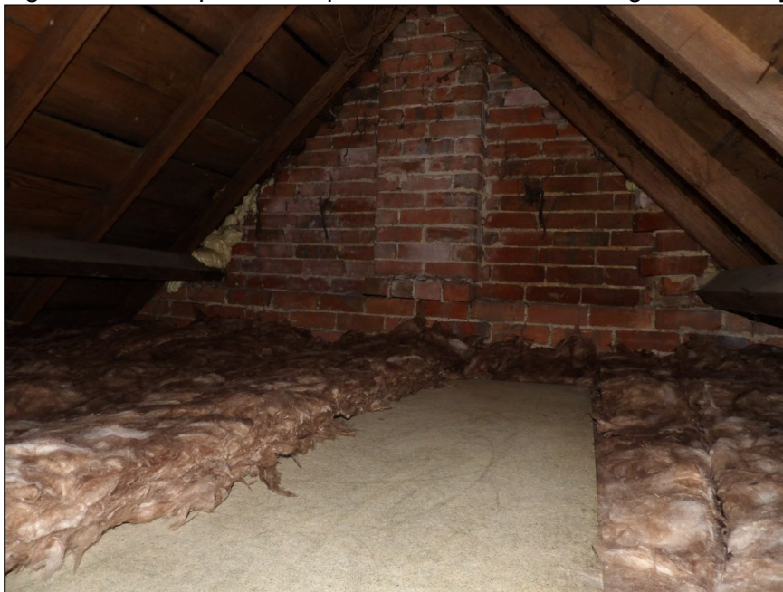
Figure 11. Example of loft space. 2 Diddenham Cottages, Grazeley. 01.10.24
