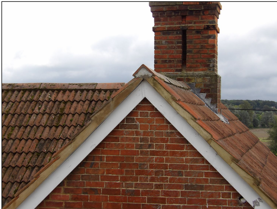
Figure 7. Example sealed verges. 2 Diddenham Cottages, Grazeley. 01.10.24
