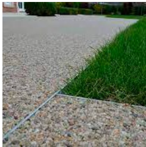
Aluminium edging to resin bound gravel
