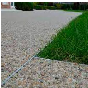
Aluminium edging to resin bound gravel
