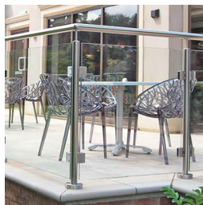
Balustrade to patio
