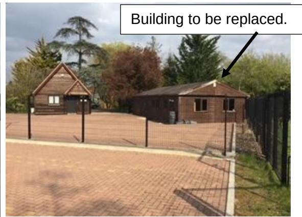
Existing ancillary buildings
