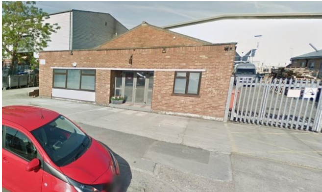
Existing store at Arkwright Road, Reading
