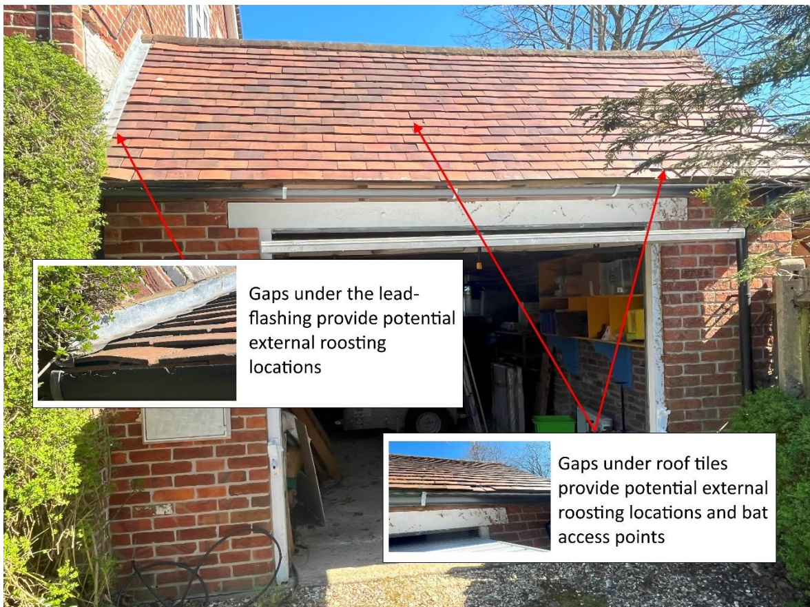
Image 4.3.2.2. Location of potential bat access points and potential external roost locations on the south-west elevation of the semi-detached garage.
