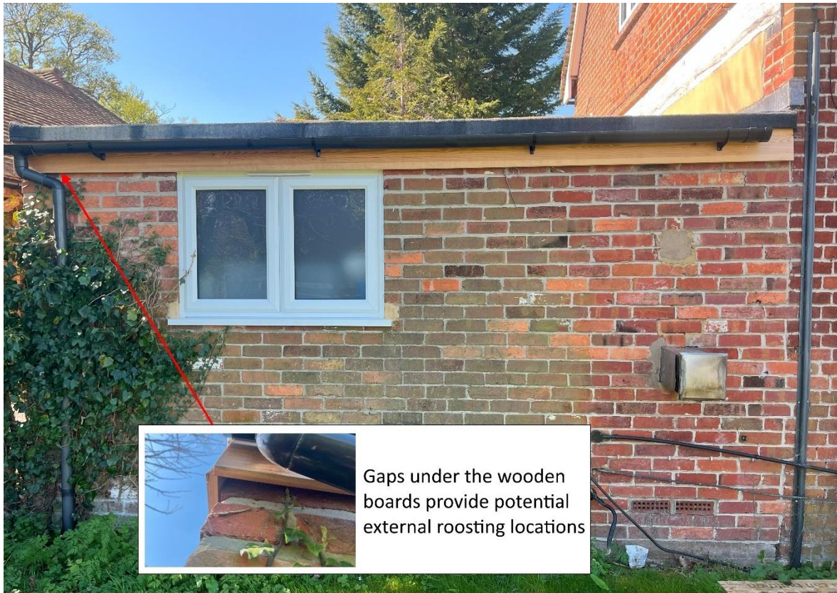
Image 4.3.2.1. Location of potential external roost locations on the north-east elevation of the semi-detached garage.
