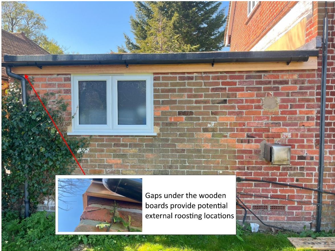
Image 4.3.2.1. Location of potential external roost locations on the north-east elevation of the semi-detached garage.
