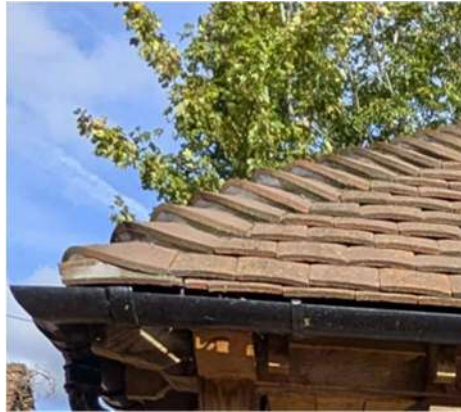
Red Clay roof tiles with bonnet hip tiles to match existing house.
