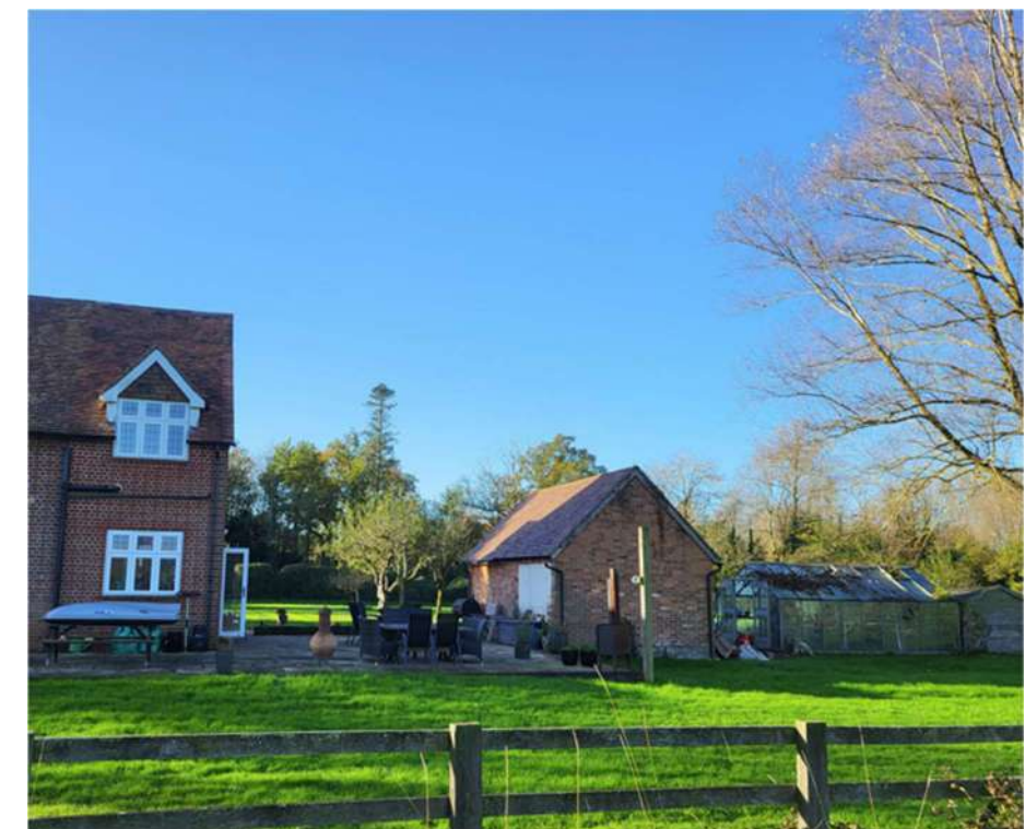
Fig. 08 Outbuildings - Brick Garage, Greenhouse & Wooden Garage from rear (looking South)
