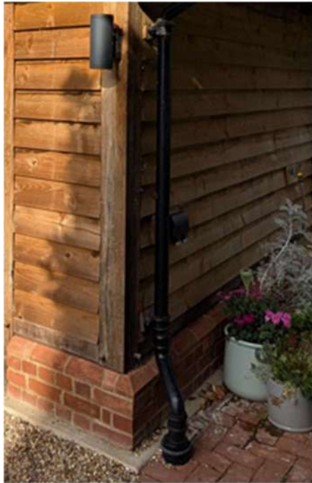
Feather-edged timber cladding to garage
