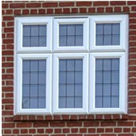
White uPVC windows to match the Existing house windows
