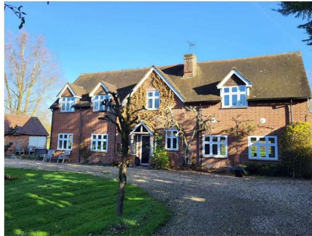
Fig. 05 Main House Front (South West) Elevation
