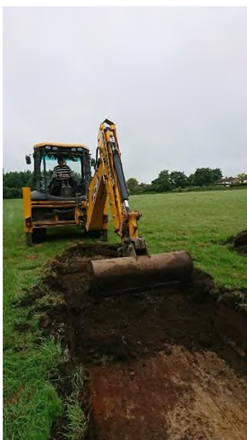
Plate 2: Trench 3 mid excavation, looking northwest
