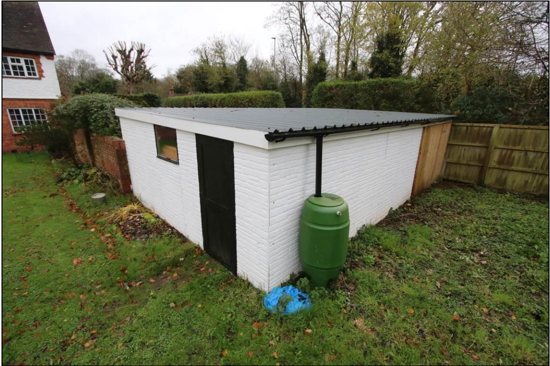
Photo 6: Single storey and pre-fabricated garage
