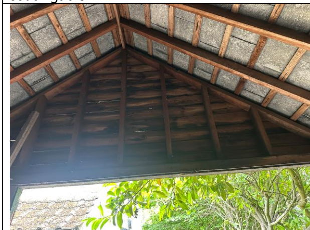
Photo 11 Garage open front
