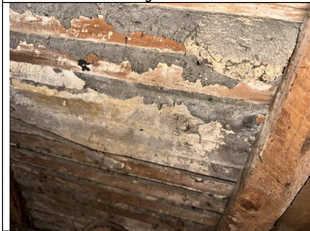
Photo 9 Plastered underside of weather boards south gable
