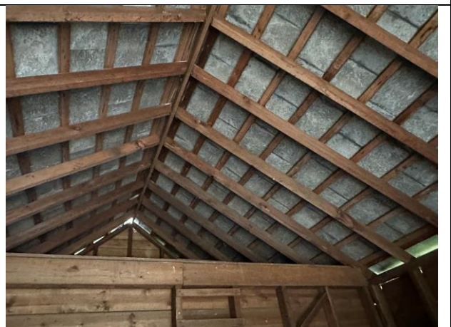
Photo 21 Garage unlined / vaulted roof
