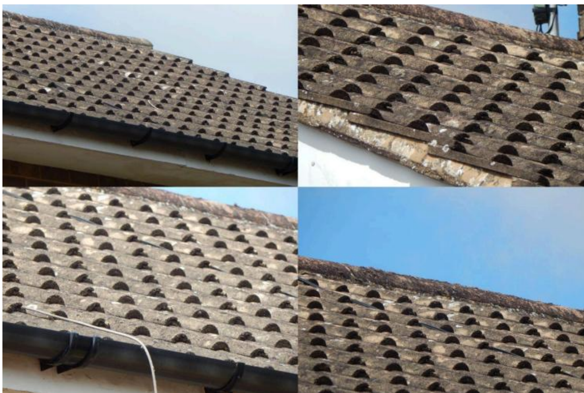
Image 6 – Close view of tiled roof coverings to demonstrate condition throughout
