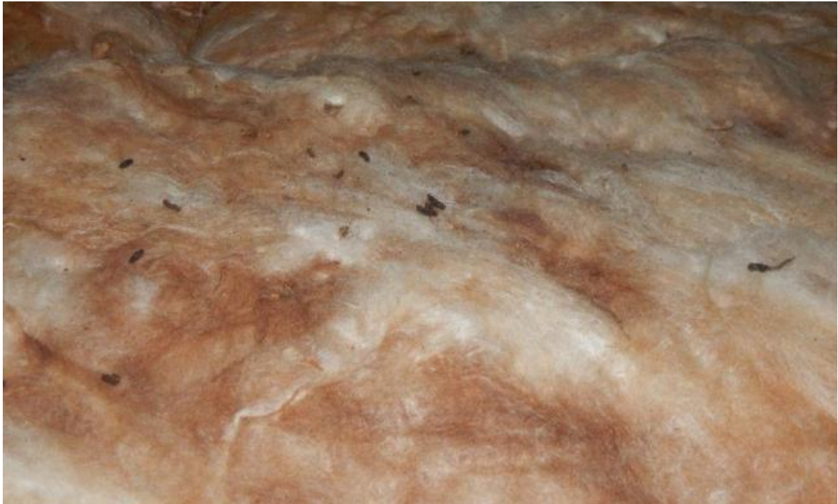
Image 9 – Small number of old droppings observed within the South section of the main roof void space
