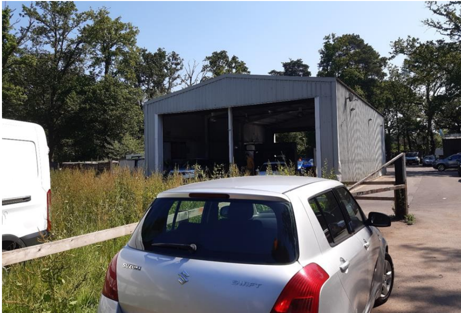
Figure 3 Taken 14.6.23 for CLUED 231266 showing blue area before change. Rear of carwash.
