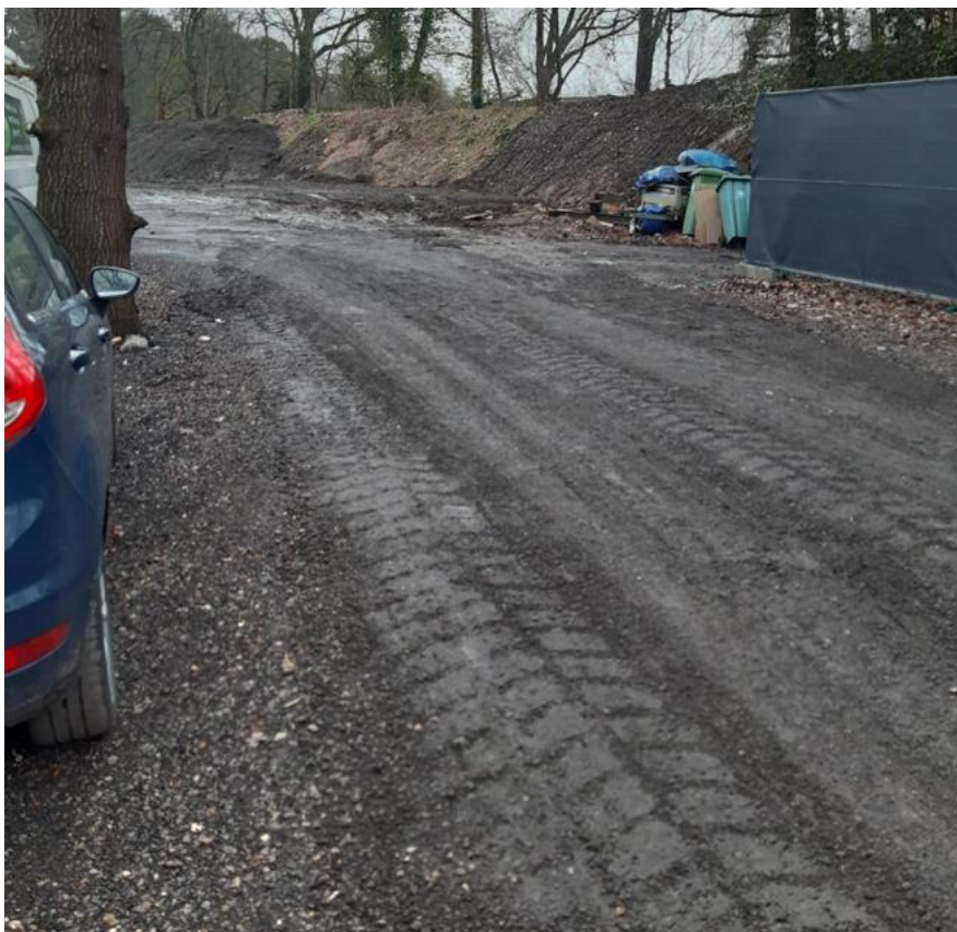
Figure 6 access way created, land cleared and fresh hard surface (in orange area)
