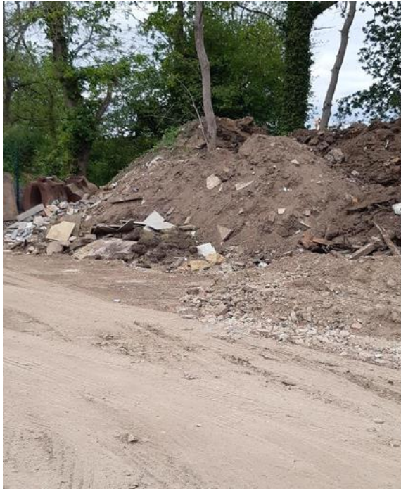
Figure 9 close up of bund around tree
