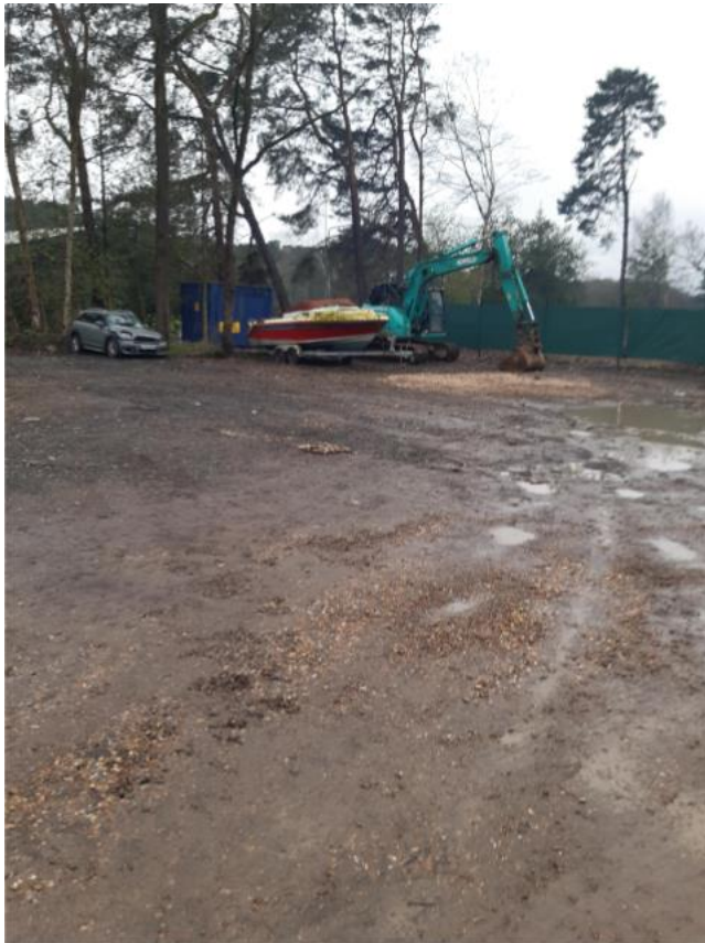
Figure 2 Blue digger in area where trees used to be and recently surfaced. This is adjacent to Notice A area to the rear and next to southern site boundary in orange area.
