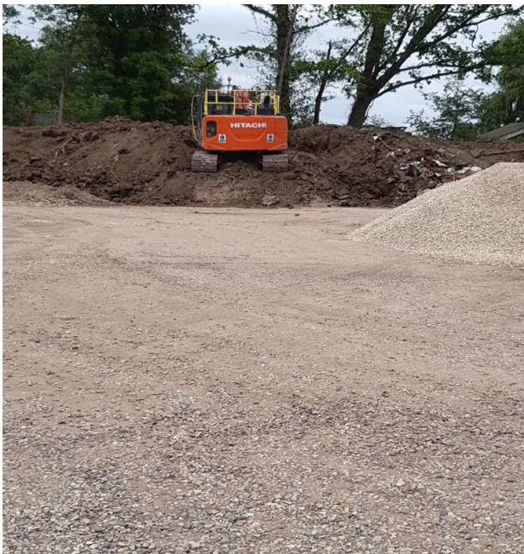
Figure 10 in process of creating bund and surfacing materials (orange area)
