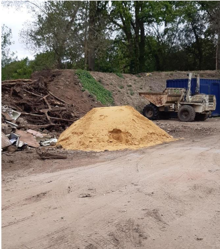
Figure 11 close up of bund
