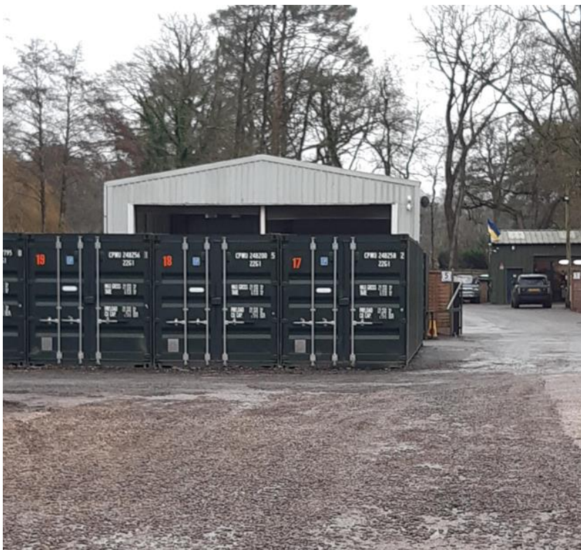
Figure 4 Blue shaded area - hard surfaced and containers, fence removed and vegetation removed
