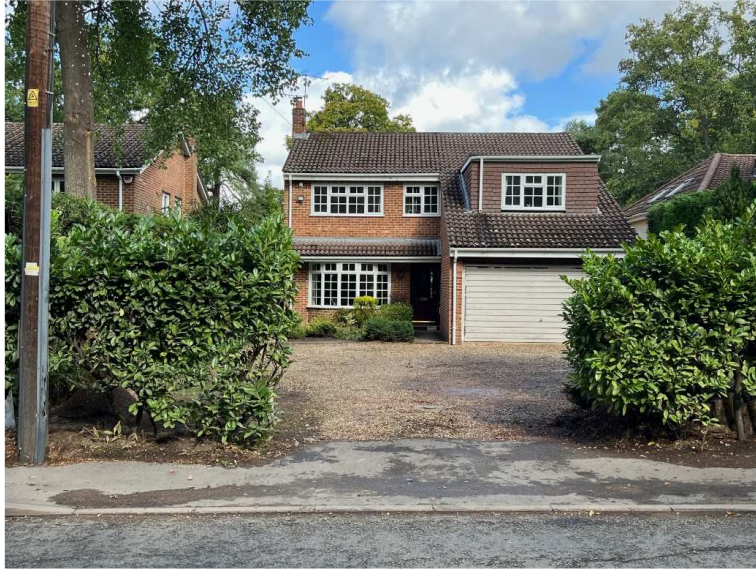
Photo of the front elevation from Nine Mile Ride
