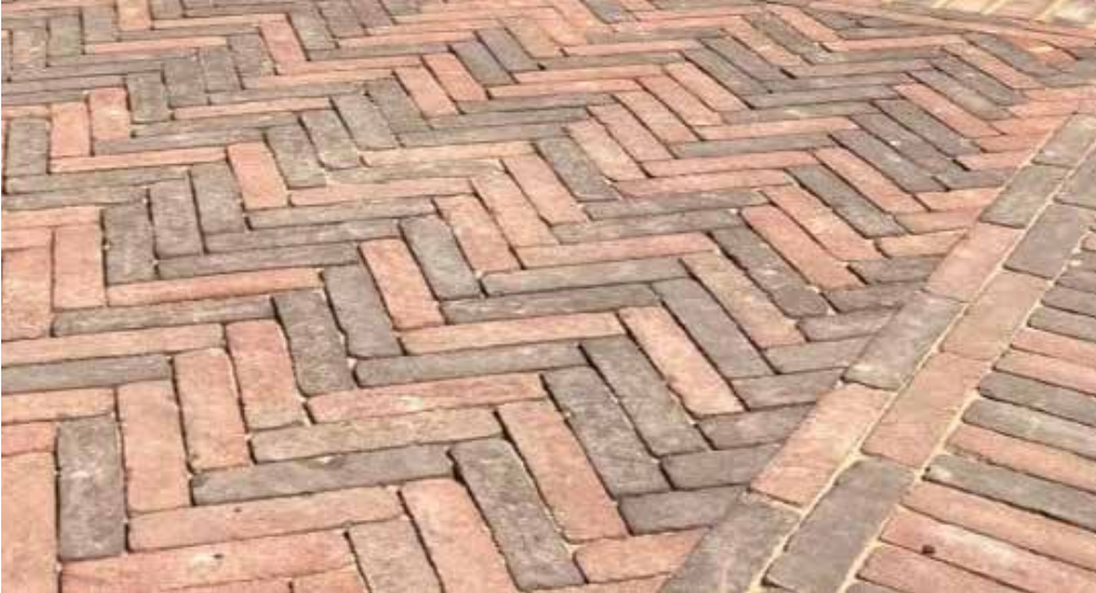
Clay pavers tying into local materiality of red brickwork
