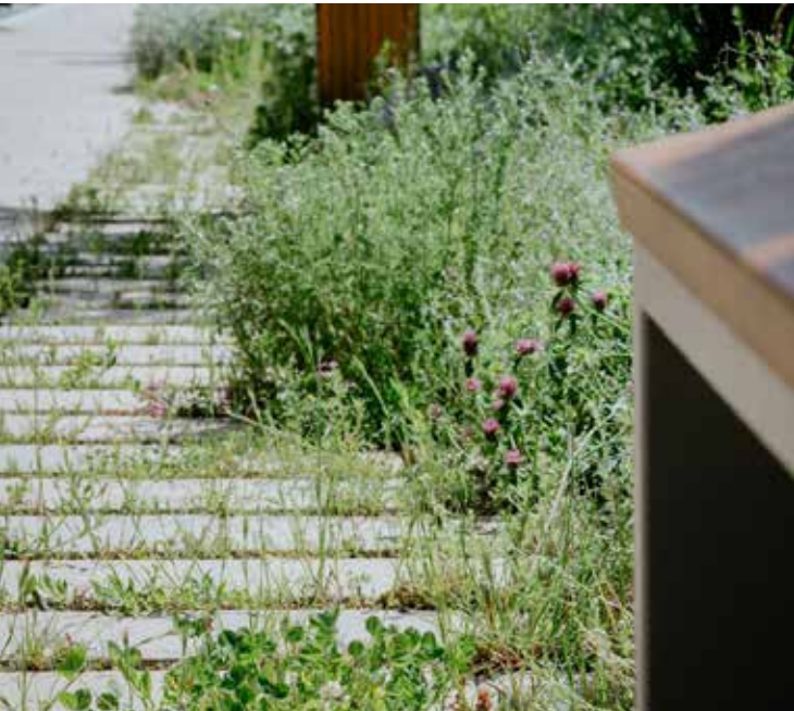
Staggered paving within existing grass
