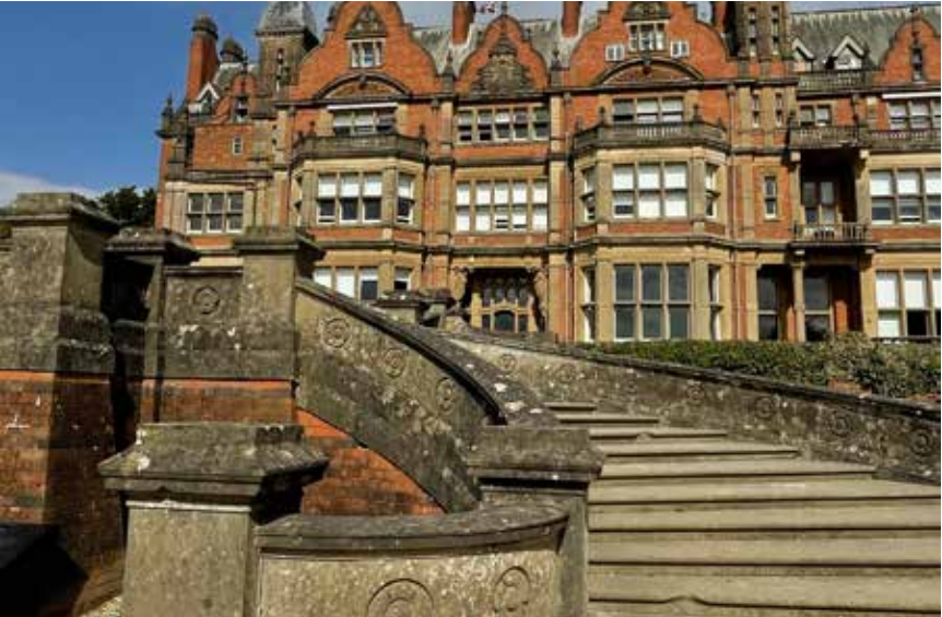
View 02 - Reddam House southern facade
