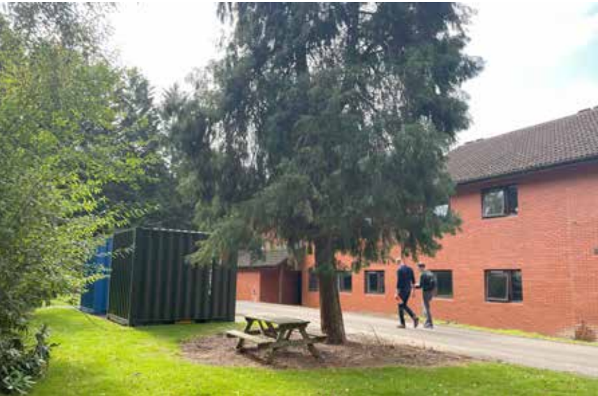
View 04 - Drake House back building
