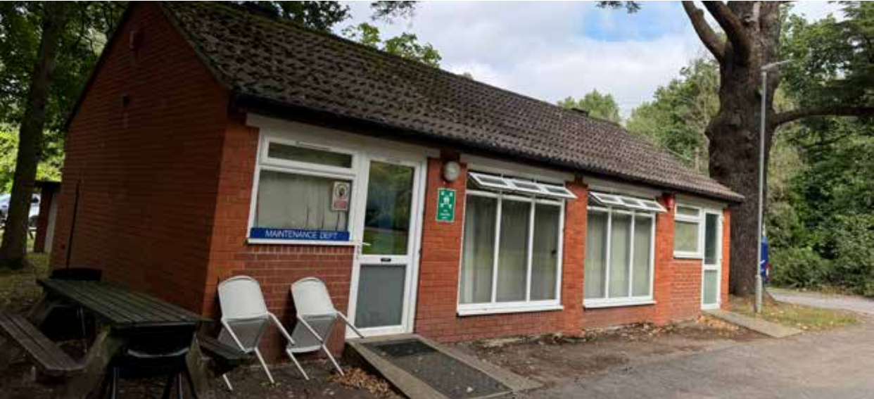
View 05 - Maintenance building
