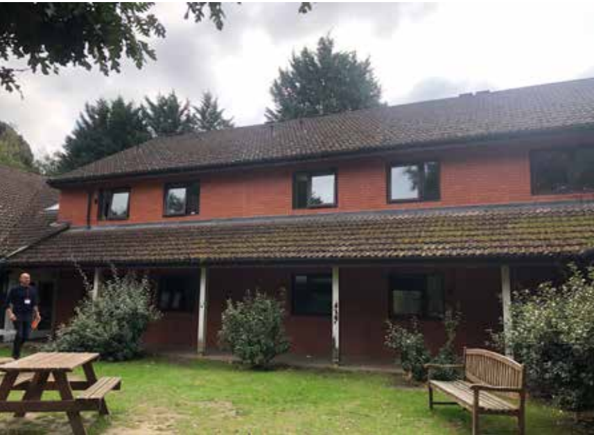
View 02 - Drake House front facade
