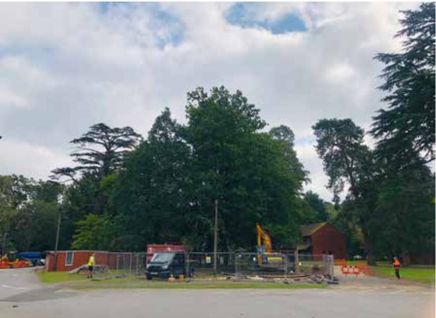
View 01 - Overview on on-going site demolition
