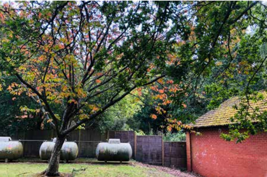
View 07 - Existing gas tank and site topography
