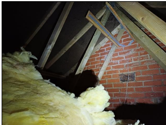
Photo 11: Internal gable end of maintenance building
