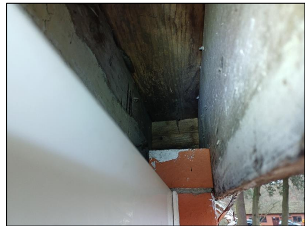
Photo 16 Medical centre gap above window - no PRF and fully explored
