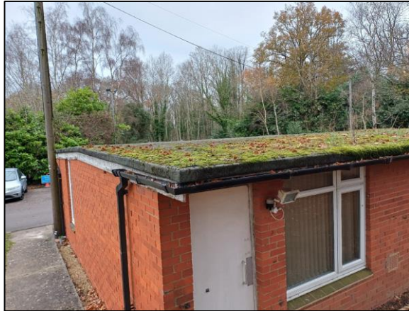
Photo 13 Medical centre roof
