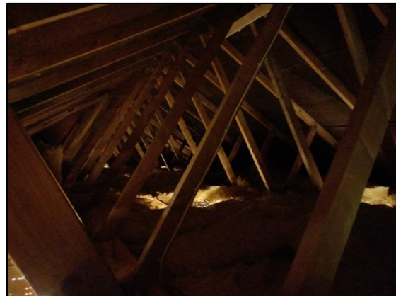
Photo 12: Loft space of maintenance building
