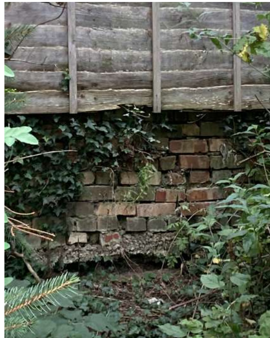
Figure. 27 | Retaining wall to be replaced. Fencing to be replaced. Northern boundary.
