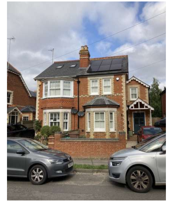
Figure. 45 | Victoria Rd - 2.5st - red brick, yellow brick quoins, slate roof.
