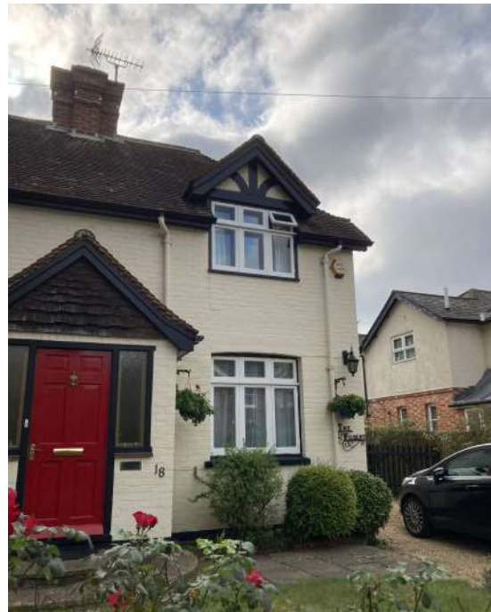
Figure. 47 | Victoria Rd - 2st - faint yellow painted brick, Tudor boarding, timber cladding, brick chimney, white UPVC window frames.
