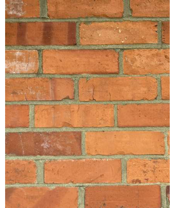
Figure. 30 | Existing nursery building brickwork facing into the site.
