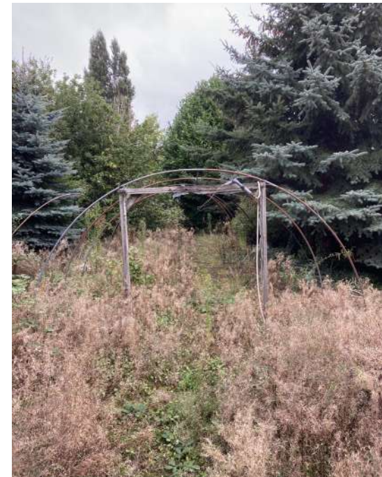
Figure. 18 | Existing structure to be removed and overgrowth.
