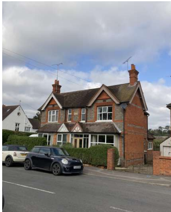
Figure. 36 | Victoria Rd - 2st - Red brick, grey brick, brick chimneys, gabling detailing, white window frames, timber detailing.
