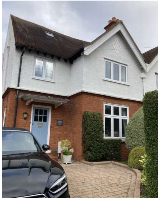
Figure. 31 | Victoria Road - 2.5st - red brick ground floor, white painted first floor.
