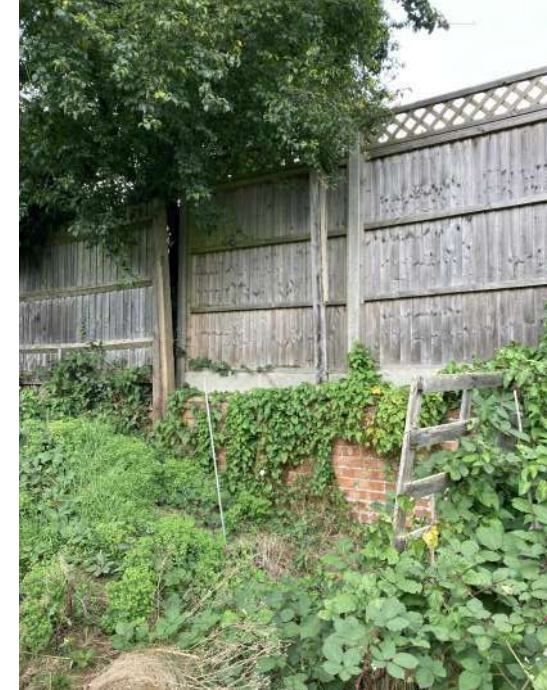
Figure. 29 | Existing close boarded fencing on top of retaining wall structure along northern boundary.
