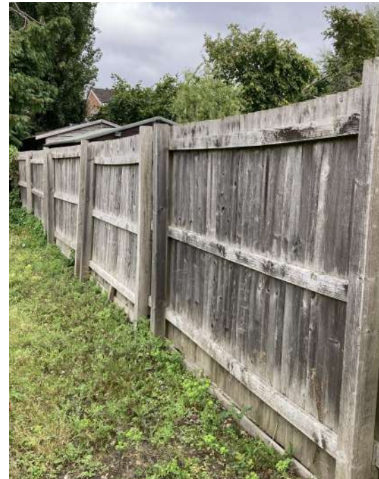
Figure. 28 | Existing close boarded fencing boundary. Eastern boundary.
