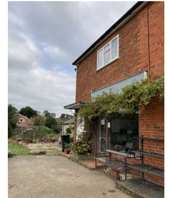
Figure. 20 | Side elevation of the nursery facing into the site.
