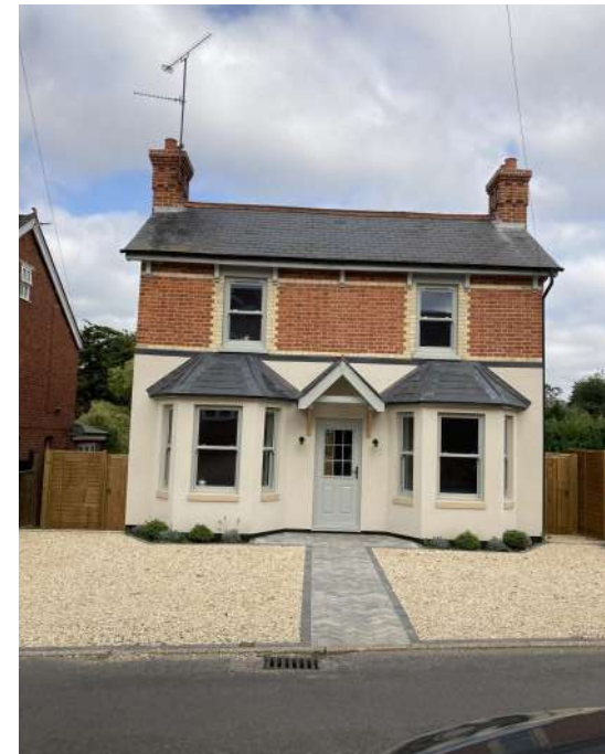
Figure. 38 | Victoria Rd - No.103 - Red brick, yellow brick details, render finished, sash window, dentils, slate roof, brick chimneys.
