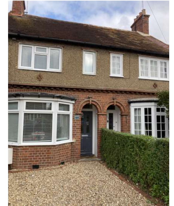
Figure. 35 | Victoria Rd - Red brick, pebble dash, clay tile, brick chimney.
