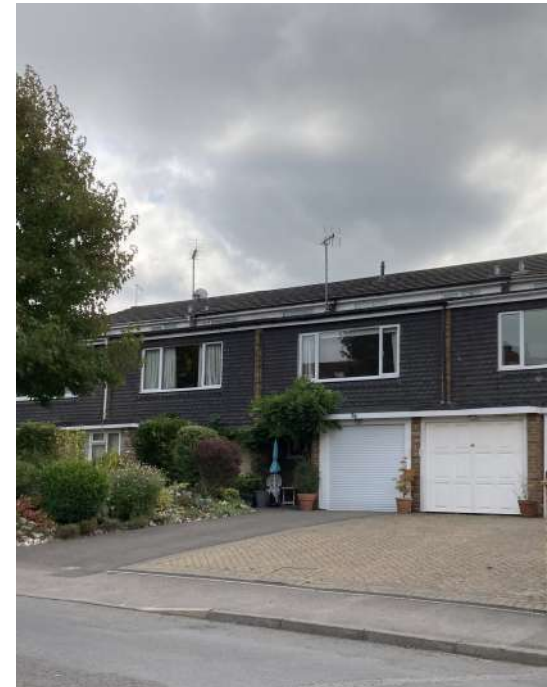
Figure. 49 | Victoria Rd - 2st - 1960's development - red brick, concrete tile hanging, concrete tiled roof, White UPVC windows, parking off main highway.
