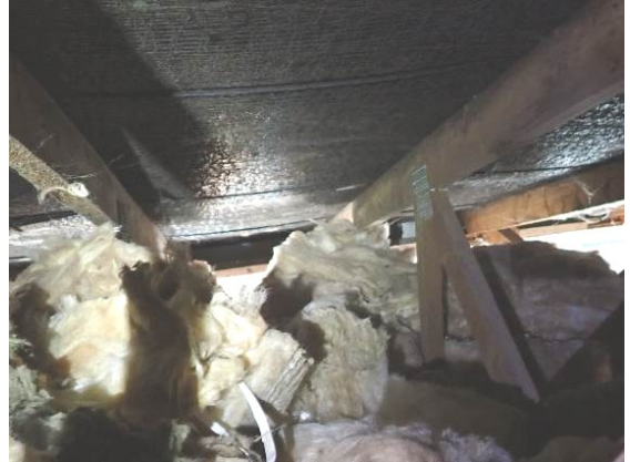
Photograph 14. Open eaves with access to the uPVC soffit.
