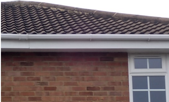
Photograph 3. Flat overlapping tiles and intact hip mortar (rear elevation).
