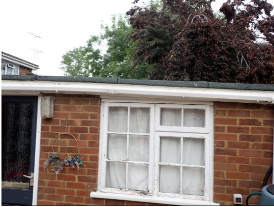
Photograph 9. Bitumen felt tight to the fascia across the flat roofed garage (southwest elevation of garage).
