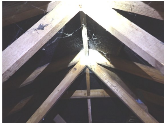
Photograph 12. Roof of trussed rafter construction.
