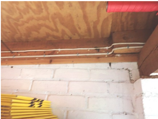
Photograph 15. Timber panels sealed to the painted brickwork (garage).
