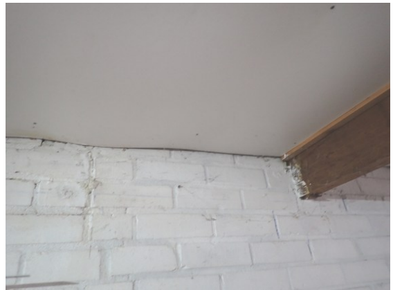
Photograph 16. Plasterboards sealed to the painted brickwork (garage).
