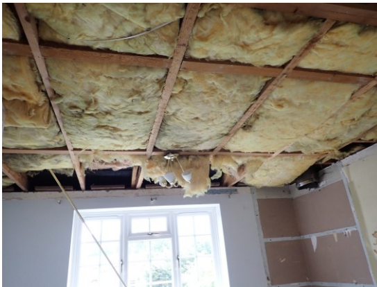
Photograph 11. Stripped ceiling with fibreglass insulation mostly remaining.
