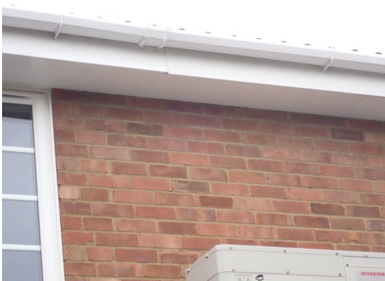
Photograph 7. uPVC soffit sealed to the brickwork (rear elevation).
