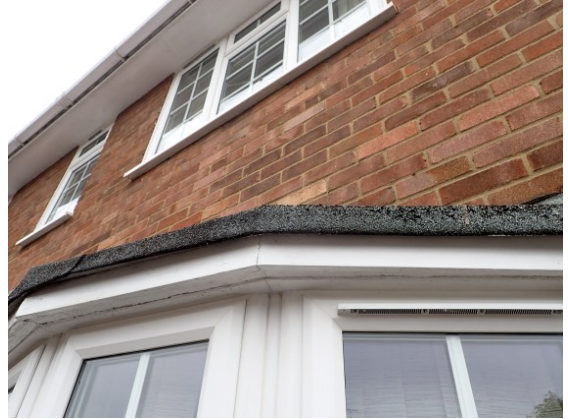
Photograph 10. Bitumen felt tight across the bay window (front elevation).
