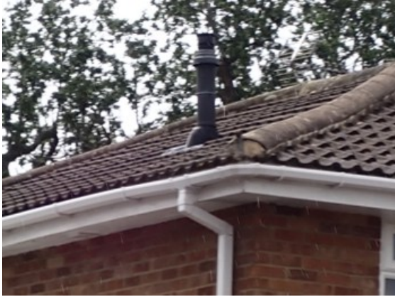
Photograph 5. Lead flashing tight to roof tiles (northeastern elevation).
