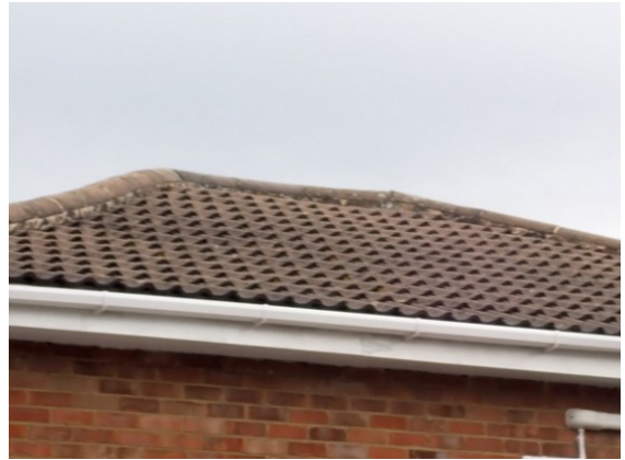
Photograph 4. Flat overlapping tiles and intact ridge and hip mortar (southwestern elevation).
