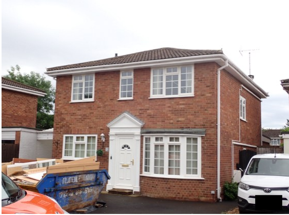
Photograph 1. Front of property viewed from the northwest.
