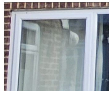
Existing UPVC white frame windows.
