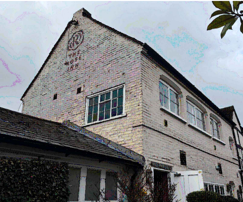
EXISTING SITE PHOTOGRAPHS
