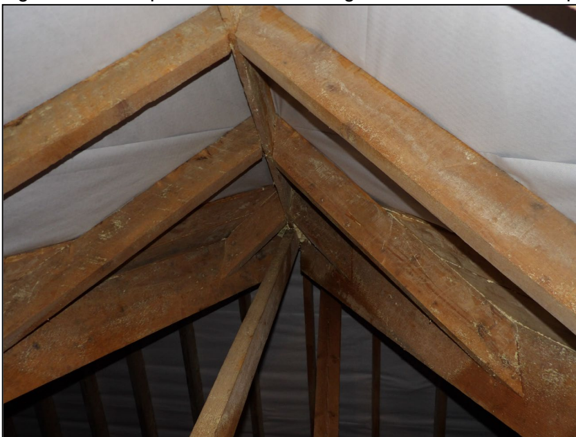
Figure 14. Example of membrane lining. 7 Pine Drive, Finchampstead. 22.04.25
