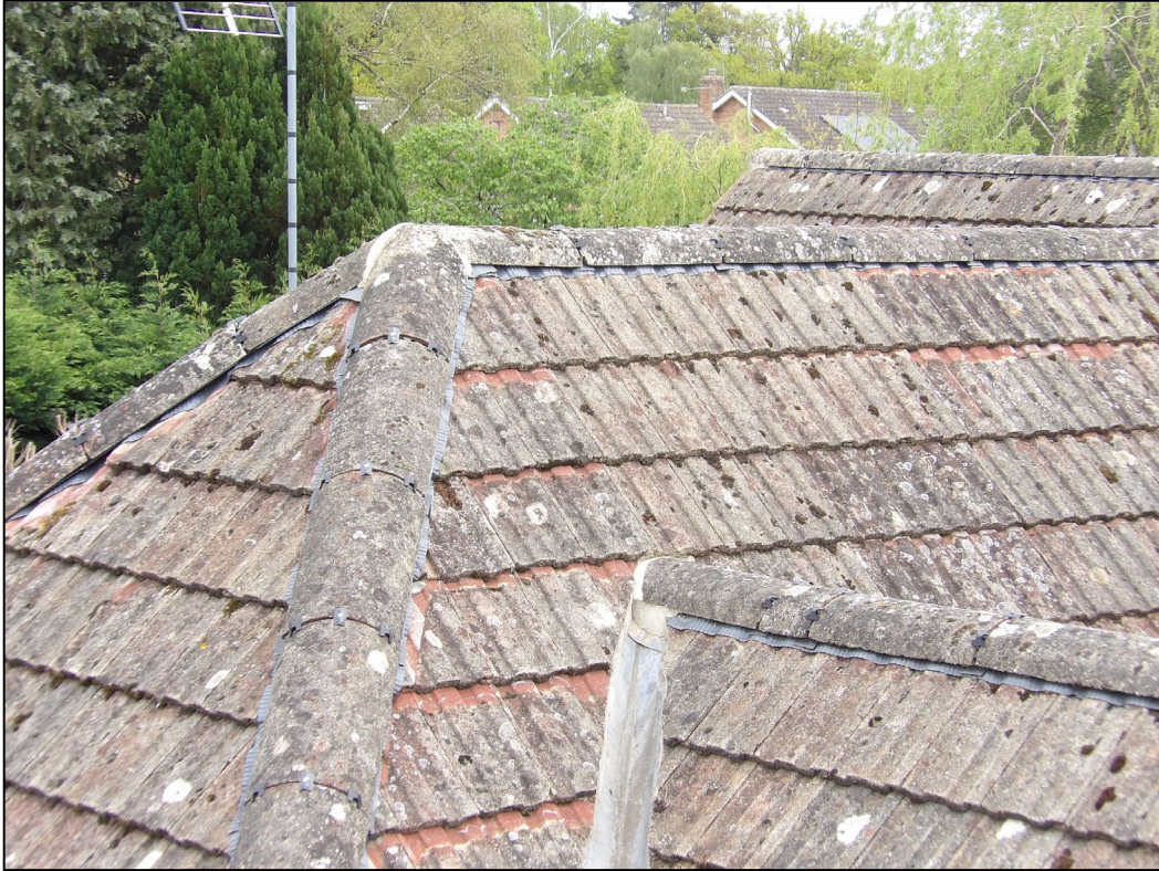
Figure 5. Example of sealed ridge/hip tiles. 7 Pine Drive, Finchampstead. 22.04.25
