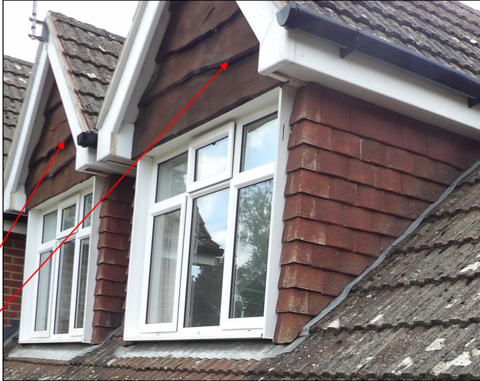
Figure 11. Hanging tiles and gaps in timber cladding on dormer windows. 7 Pine Drive, Finchampstead. 22.04.25
