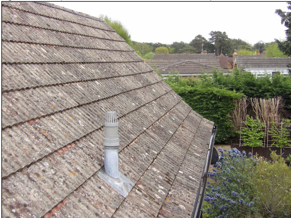
Figure 4. Example of roof tiles. 7 Pine Drive, Finchampstead. 22.04.25
