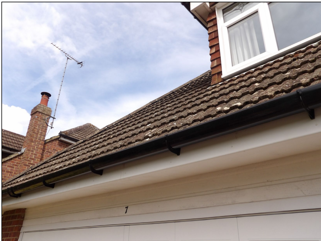
Figure 8. Sealed fascias and up-and-over garage door. 7 Pine Drive, Finchampstead. 22.04.25
