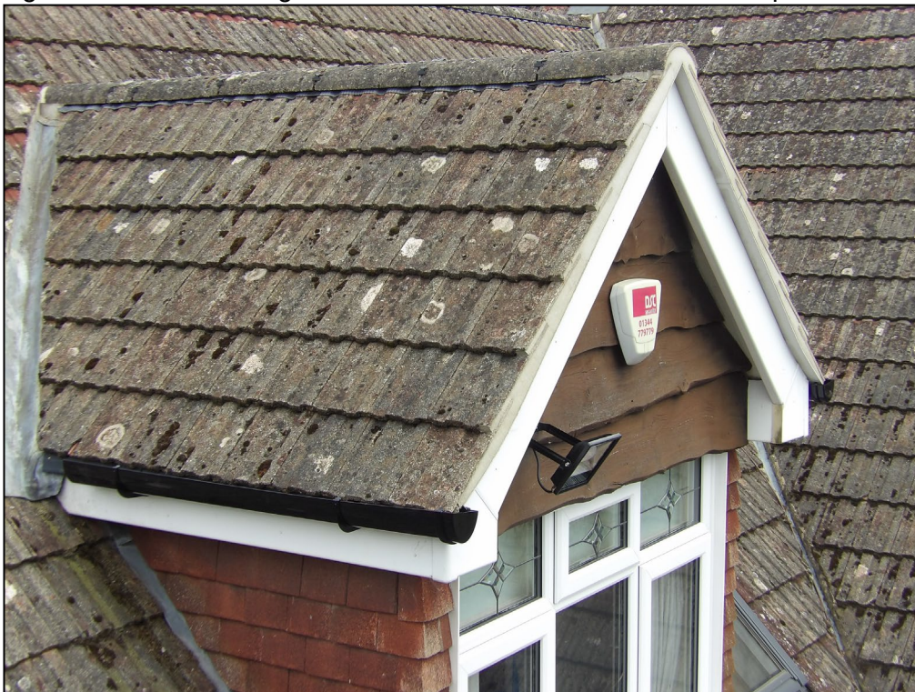
Figure 10. Tiles covering dormer windows. 7 Pine Drive, Finchampstead. 22.04.25
