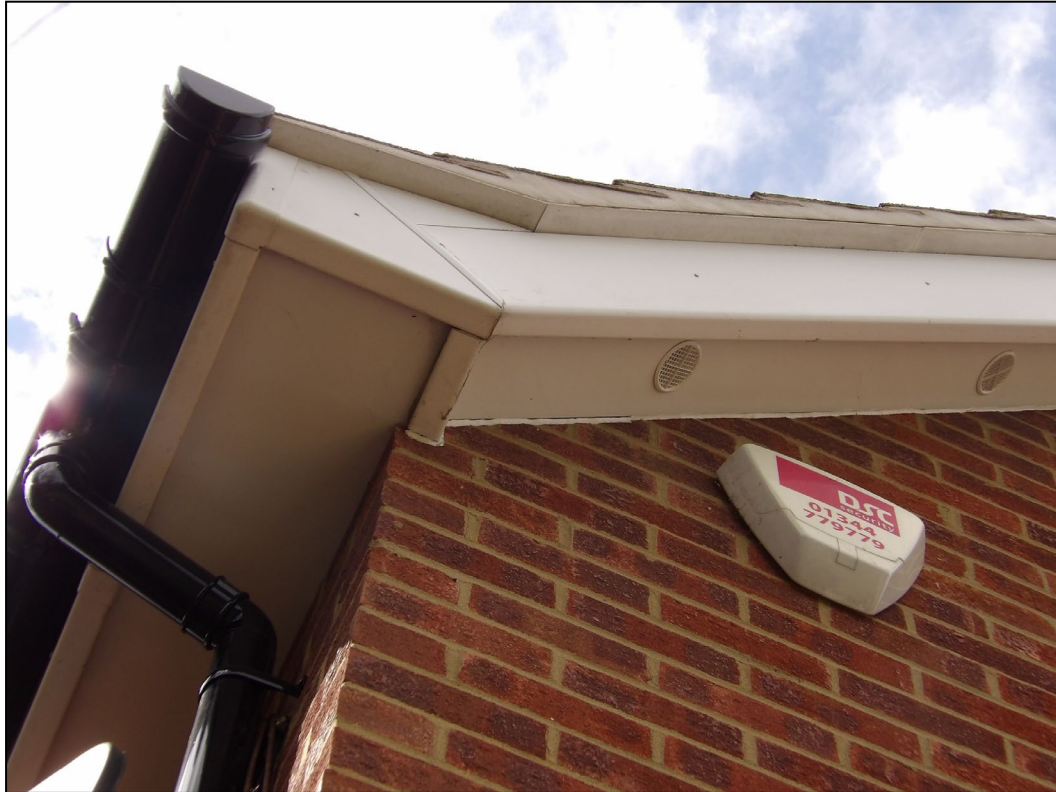
Figure 7. Example of soffits/fascias. 23b Pine Drive, Finchampstead, 02.07.24
