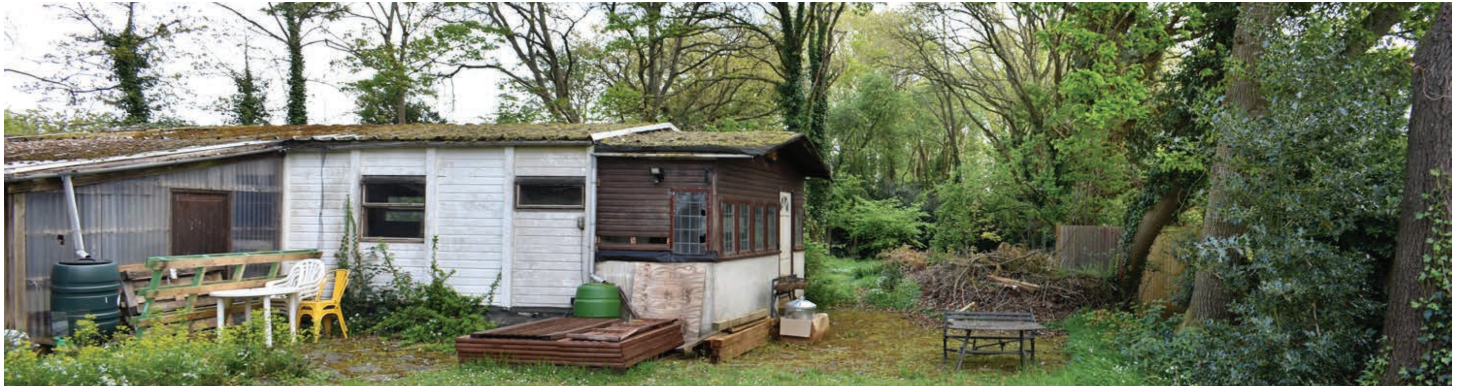
Photograph A View looking east towards existing building
