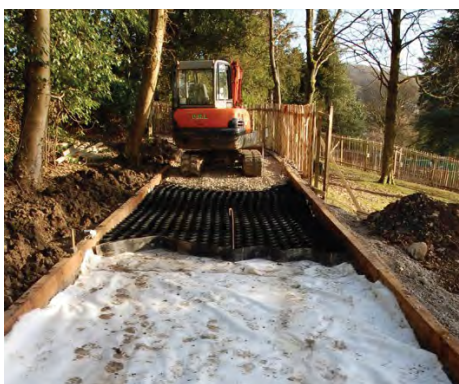
Fallbarrow Park, Windermere: CellWeb TRP® Installation
