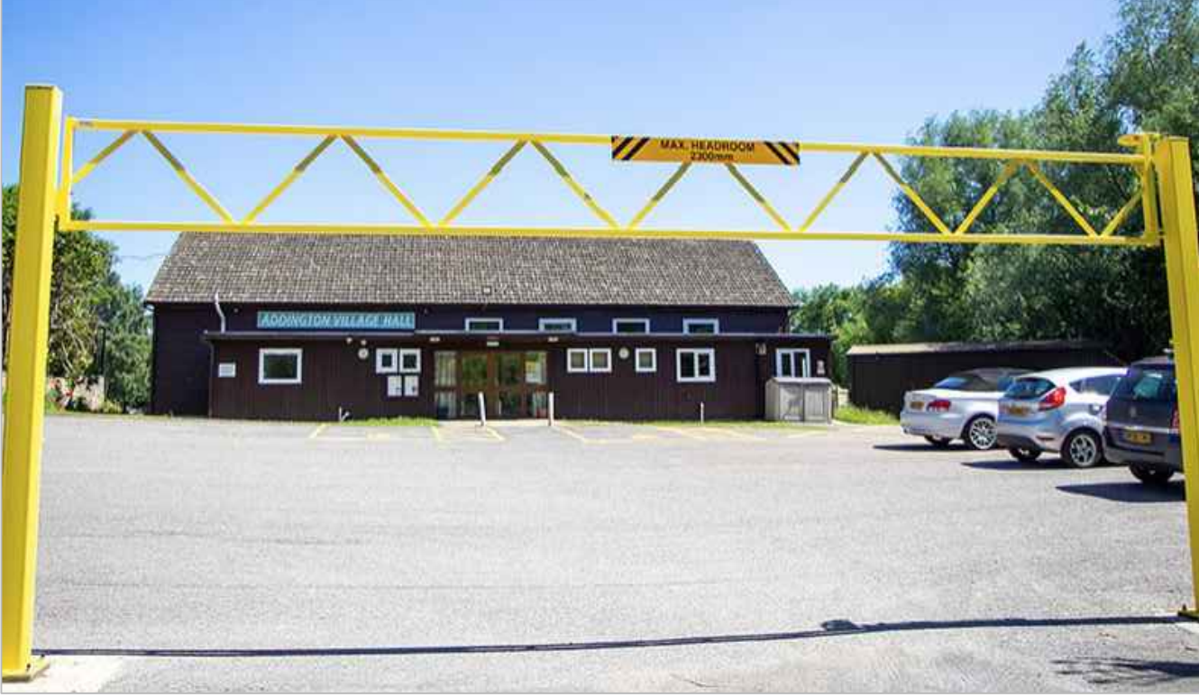
Vehicle Height Restriction Barrier
