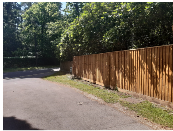
Figure 4 Site visit photo towards Wellingtonia Avenue taken 22 June 2026
