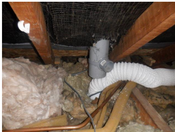
Photograph 12. Gap around a flue pipe.
