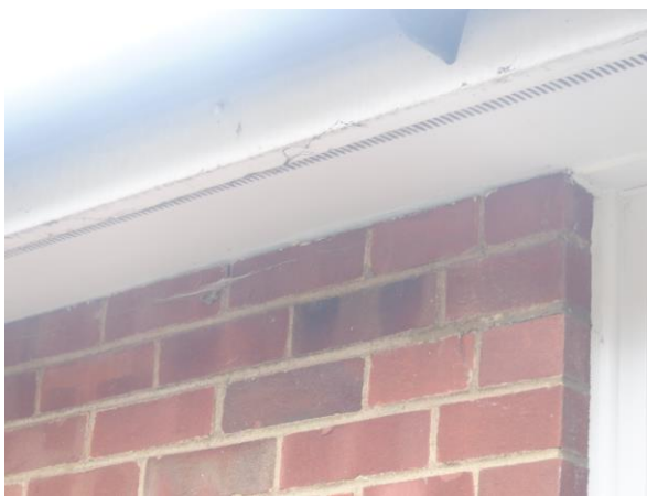
Photograph 8. Vented uPVC soffits tight around the eaves.
