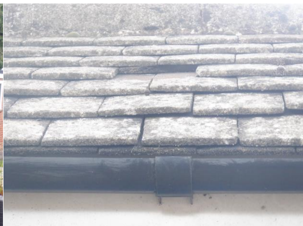
Photograph 10. Broken roof tile to the front of the garage.
