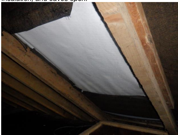
Photograph 13. Small section of roof with breathable roofing membrane.
