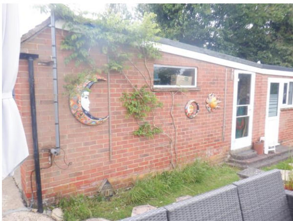
Photograph 9. Garage with a flat bitumen lined roof and uPVC barge boards.
