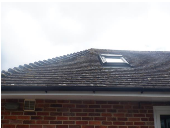
Photograph 4. Flat roof tiles in place and intact, and ridge and hip tiles fully mortared.
