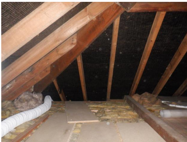
Photograph 11. Roof void boarded with fibreglass insulation, and eaves open.
