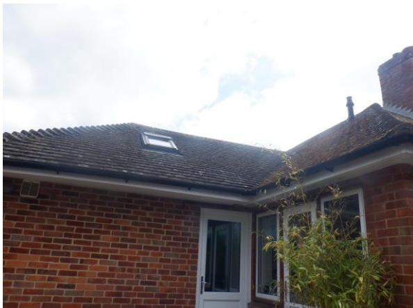
Photograph 7. Lead flashing tight around the skylight and chimney.
