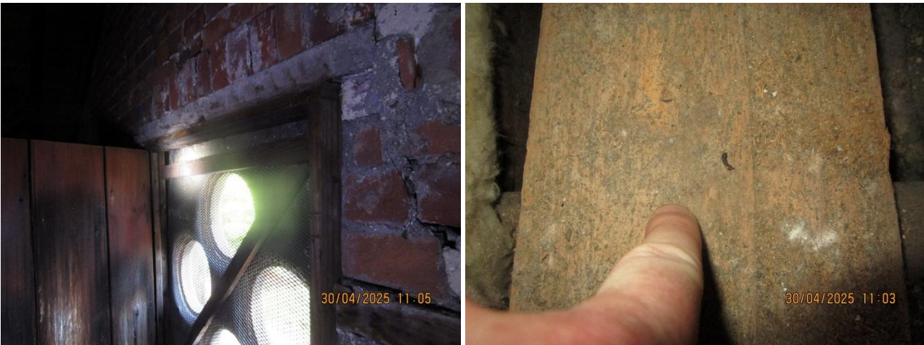
Photo 11 – Round headed window at the gable end, with gaps between the mesh and brickwork, and, Photo 12 – Scattered bat dropping within the loft
