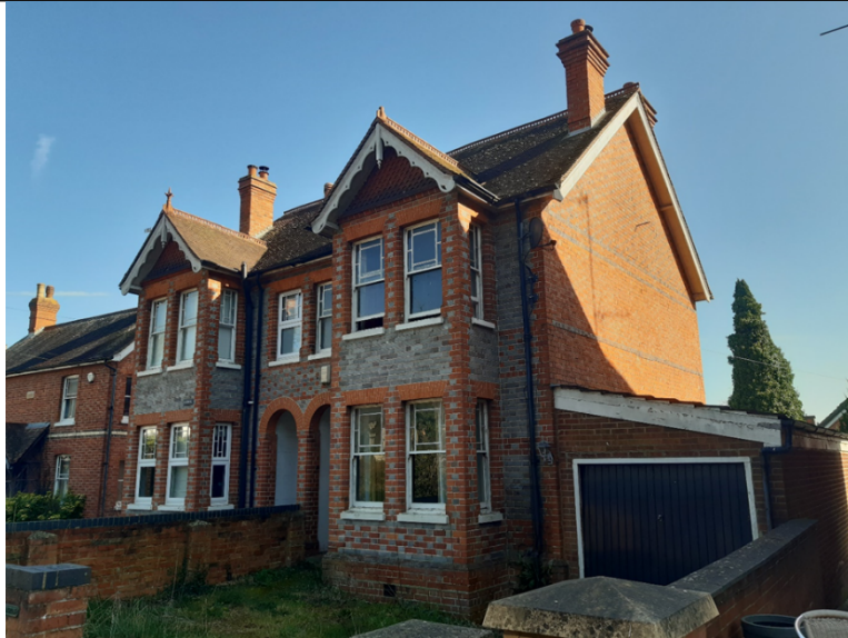
Figure 1 Front and side of Arlington as seen from the highway.
