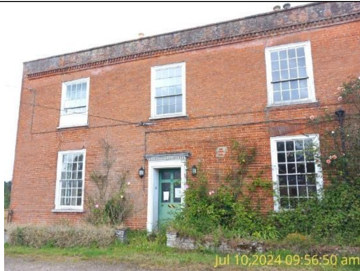
Figure 1: B1 – Northeast elevation.
