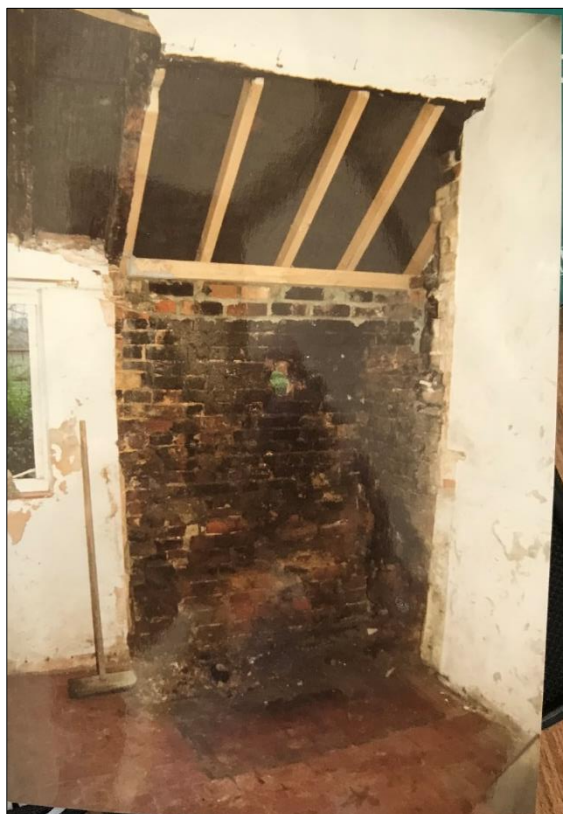
Fig. 15a. Rear room with fireplace removed and late C20 door.
