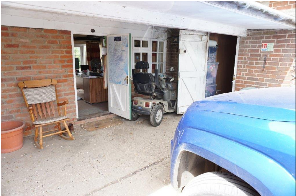
Fig. 17. Late C20 canopy, windows, doors and wall to east elevation.
