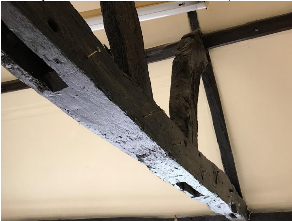
Fig. 18b. Trusses formed of re-used timbers in former office/open shed.
