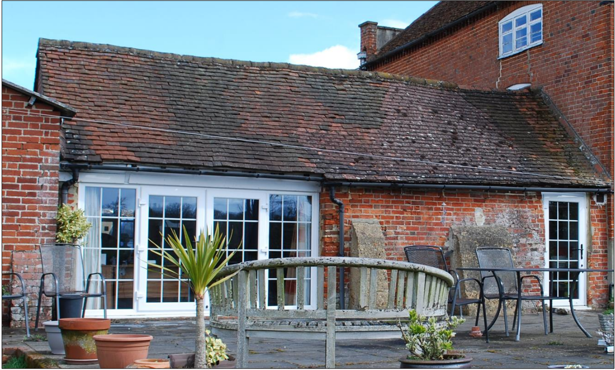
Fig. 16. Garden elevation. Late C20 windows, doors and canopy.
