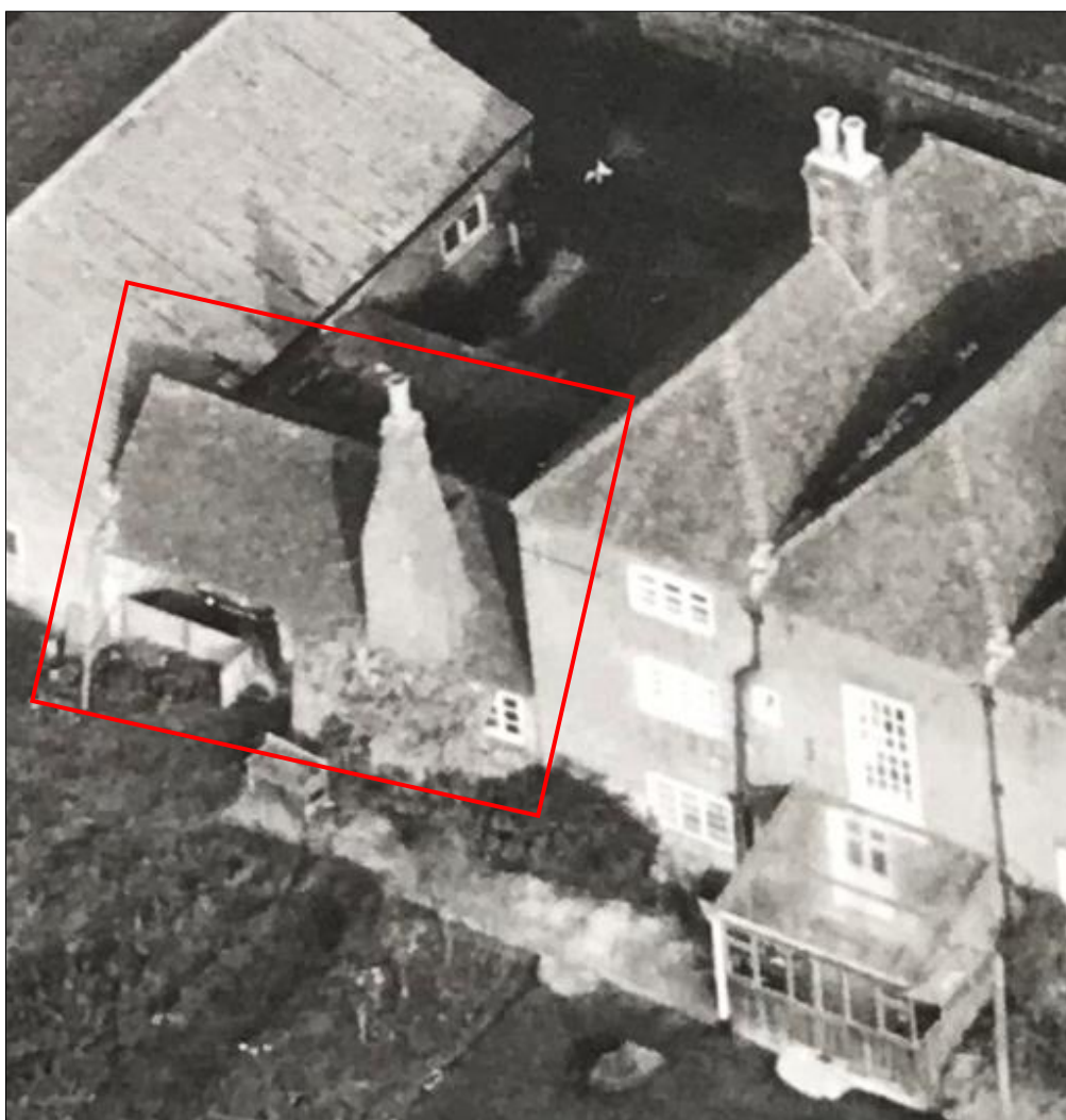
Fig. 14. Late C20. Aerial view showing stack and open shed.
