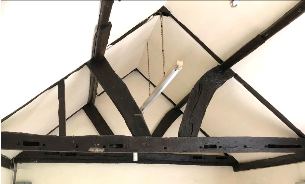
Fig. 18a. Trusses formed of re-used timbers in former office/open shed.
