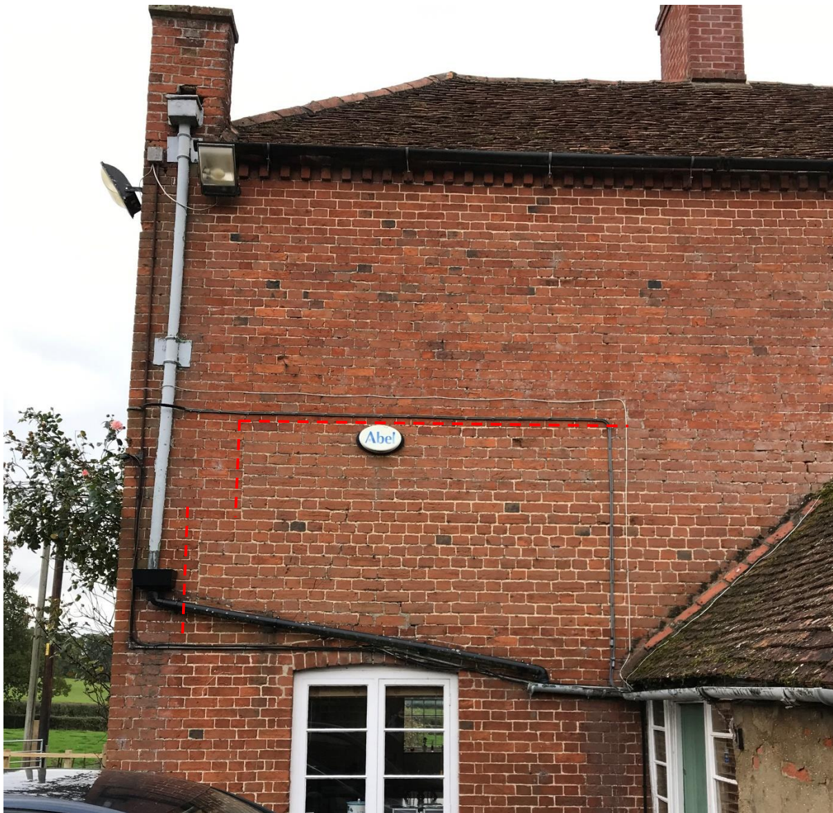
Fig. 3. Straight joints/differences in brickwork on the north elevation.
