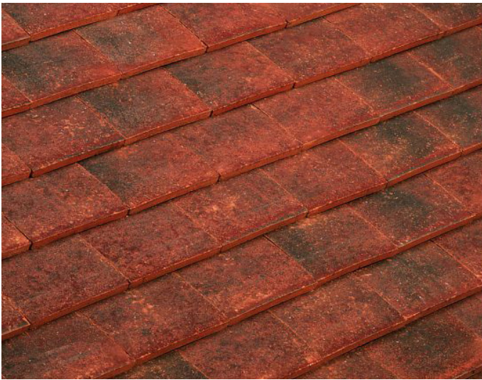
Roof - Red Clay Tile
