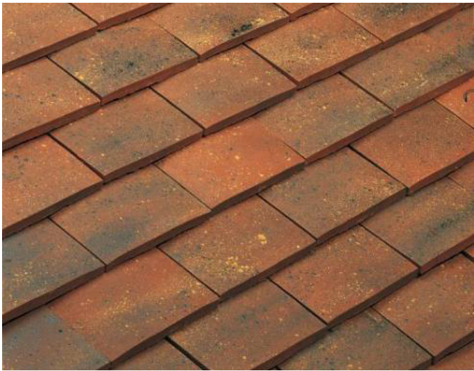
Roof - Orange Clay Tile
