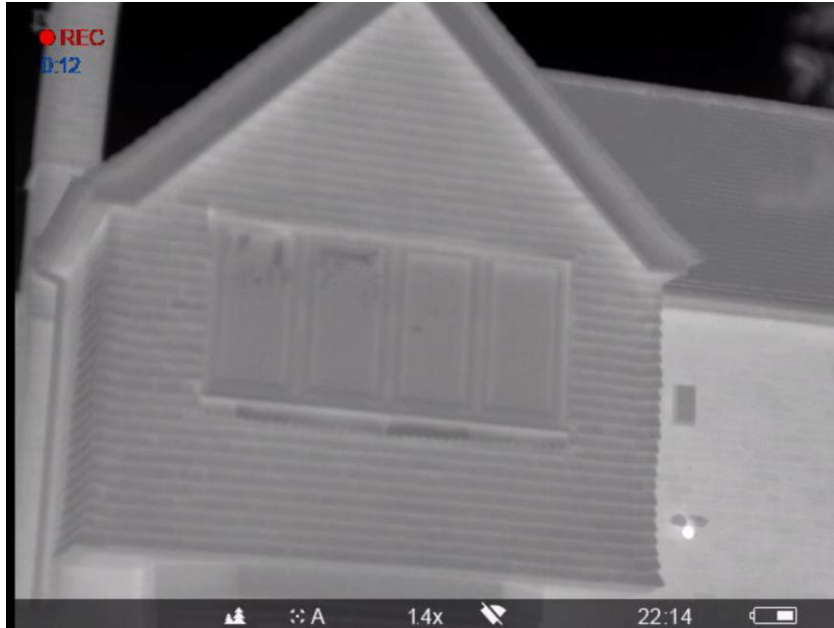
Pulsar Hellion XP28 at Surveyor Location 1.
