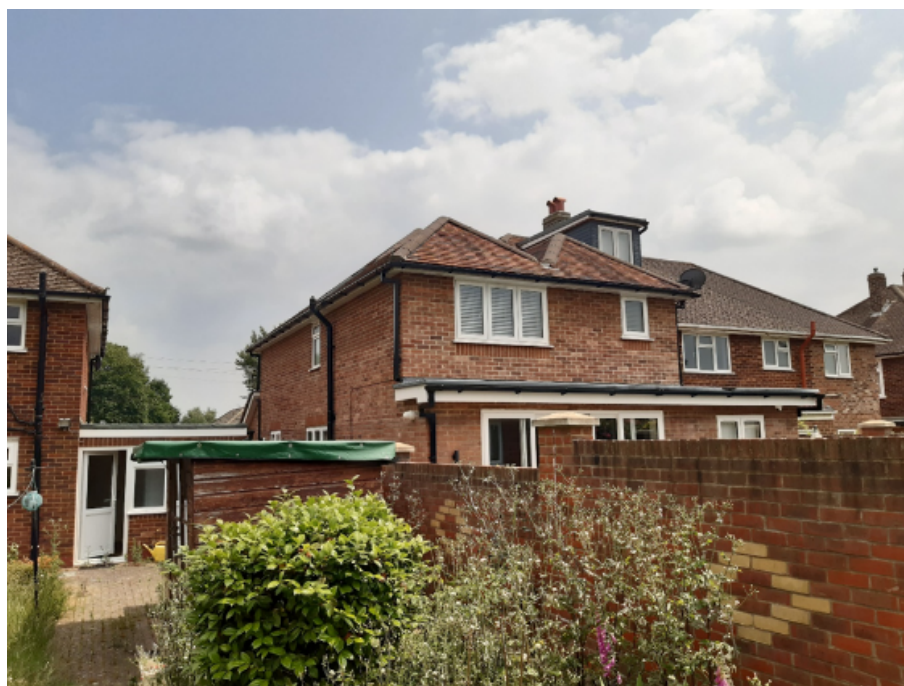
Figure 4 Rear view of no. 16 from 14 Selsdon Avenue.
