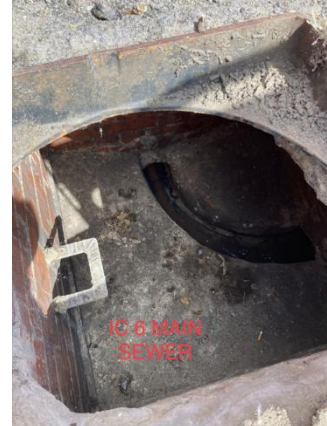
Photo 39: IC 6 Main sewer
