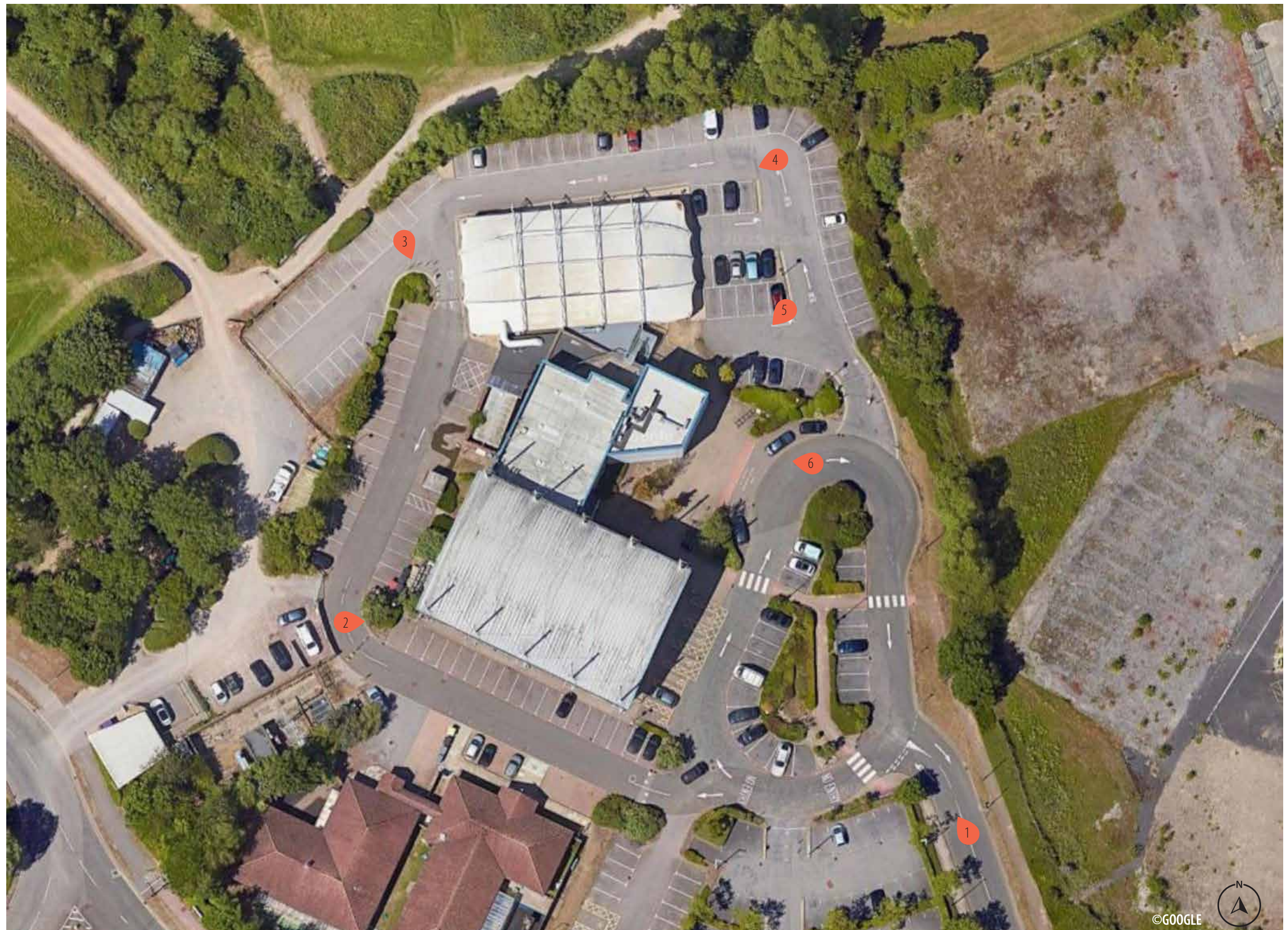
Fig. 3 Site Aerial Photograph
