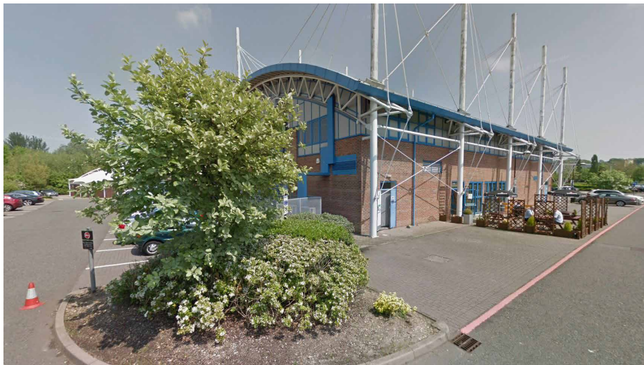
Photo 2 View 2 - Side of existing club
