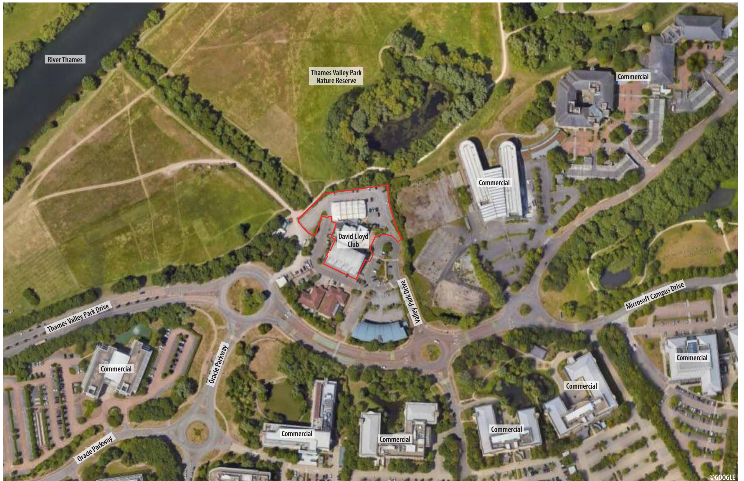
Fig. 1 Site Aerial View
