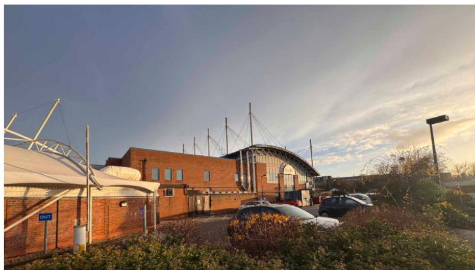
Photo 3 View 3 - Rear of existing club
