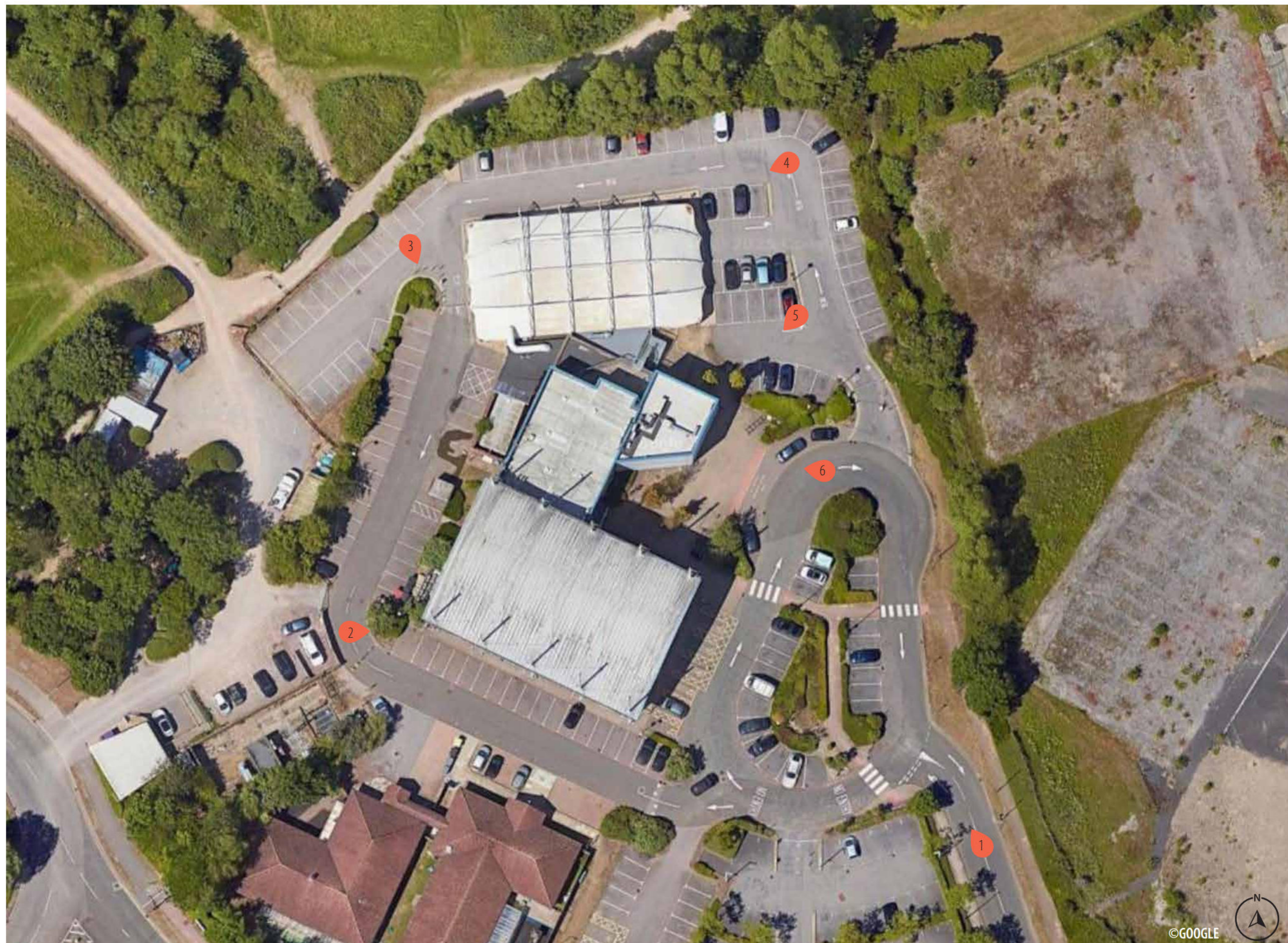
Fig. 3 Site Aerial Photograph
