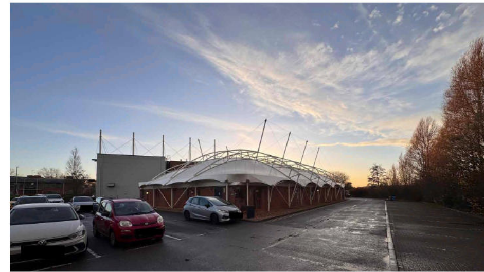
Photo 4 View 4 - Rear of existing pool
