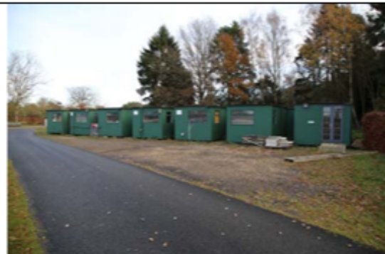
Plate 9 – Line of seven former site cabins positioned behind polo practice ground with hard standing to their front.
