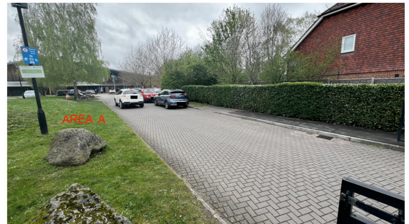
Plate 4 View of raised landscaping and planting to left of principal entrance. Note unallocated, random parking adjacent to this area, restricting visibility and access at this point. Pedestrian footpath abutting vehicular access.
