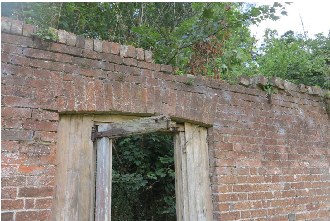
Plate 16. The walled garden (doorway in the southern wall) (September 2025)
