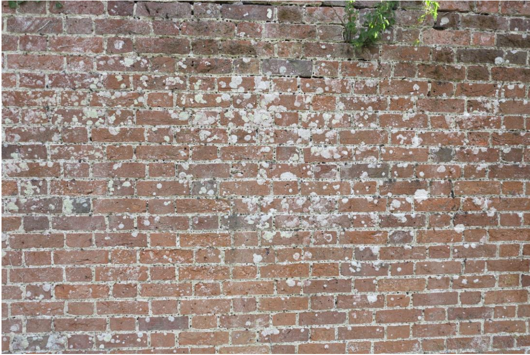
Plate 17. The walled garden (detail of southern wall) (September 2025)
