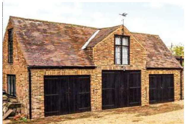
Figure 11. Existing garage front elevation
