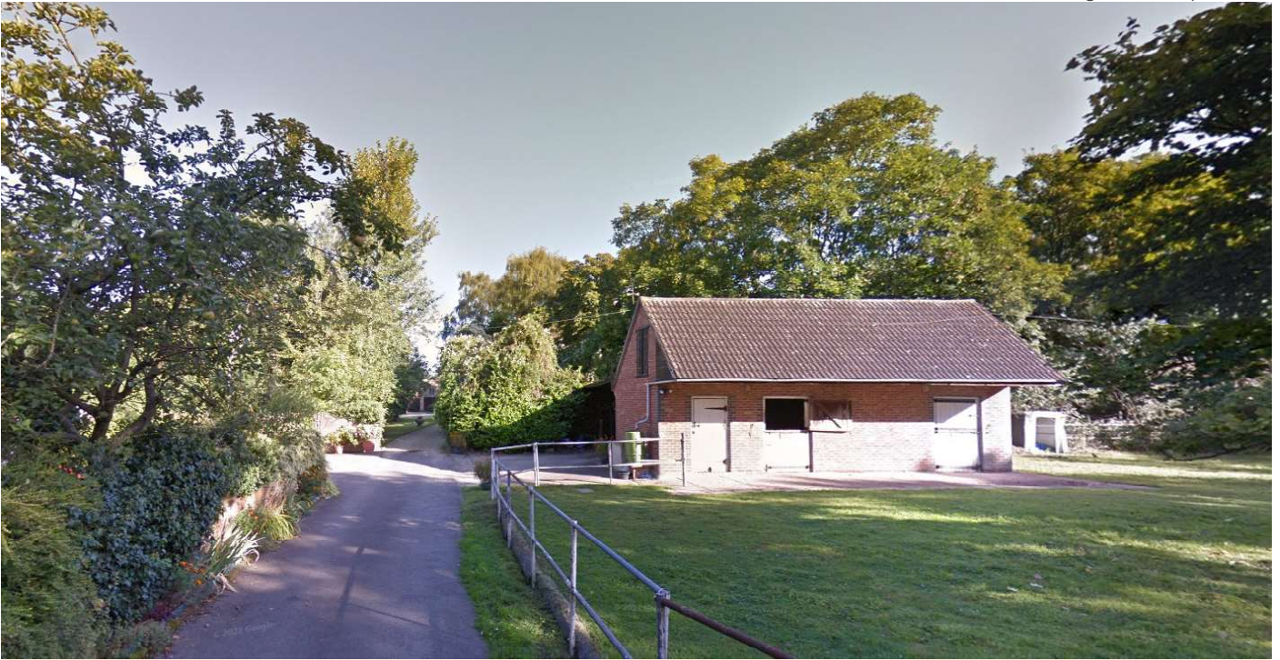
Figure 7. View up driveway to High Chimneys - Image taken from Google Maps
