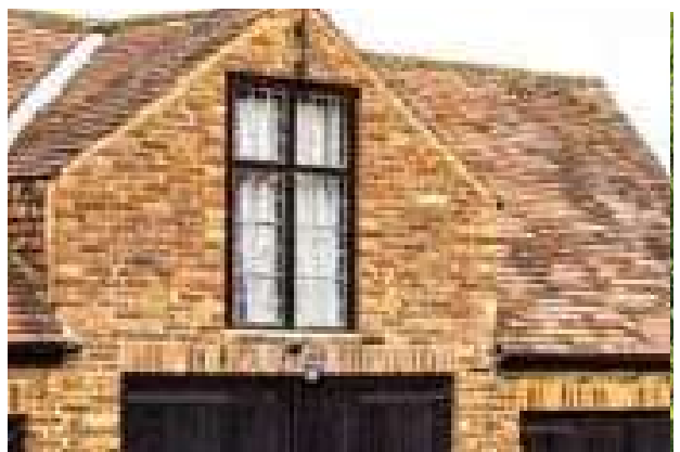
Figure 13. Black timber leded windows to garage
