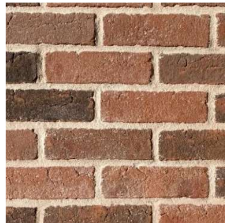
Red Multi/Brown Brickwork
