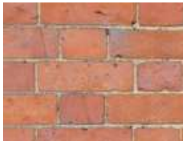
Red brickwork Flemish Bond
