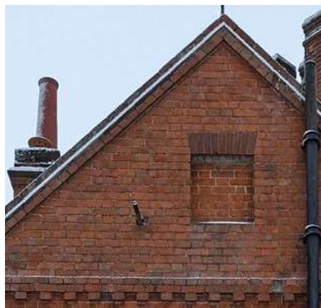
Gable Brick Detailing
