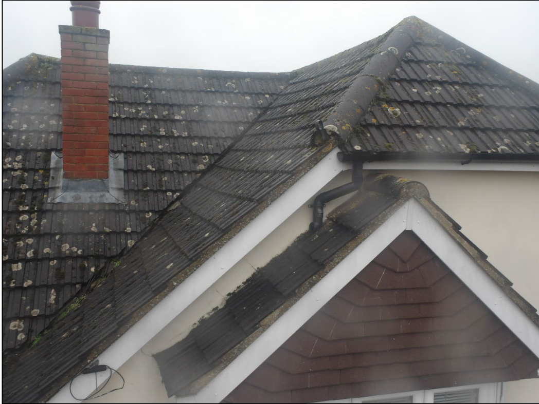
Figure 5. Example of close-fitting/sealed ridge/hip tiles/valleys and verges. 52 Oatlands Road, Shinfield. 08.02.24
