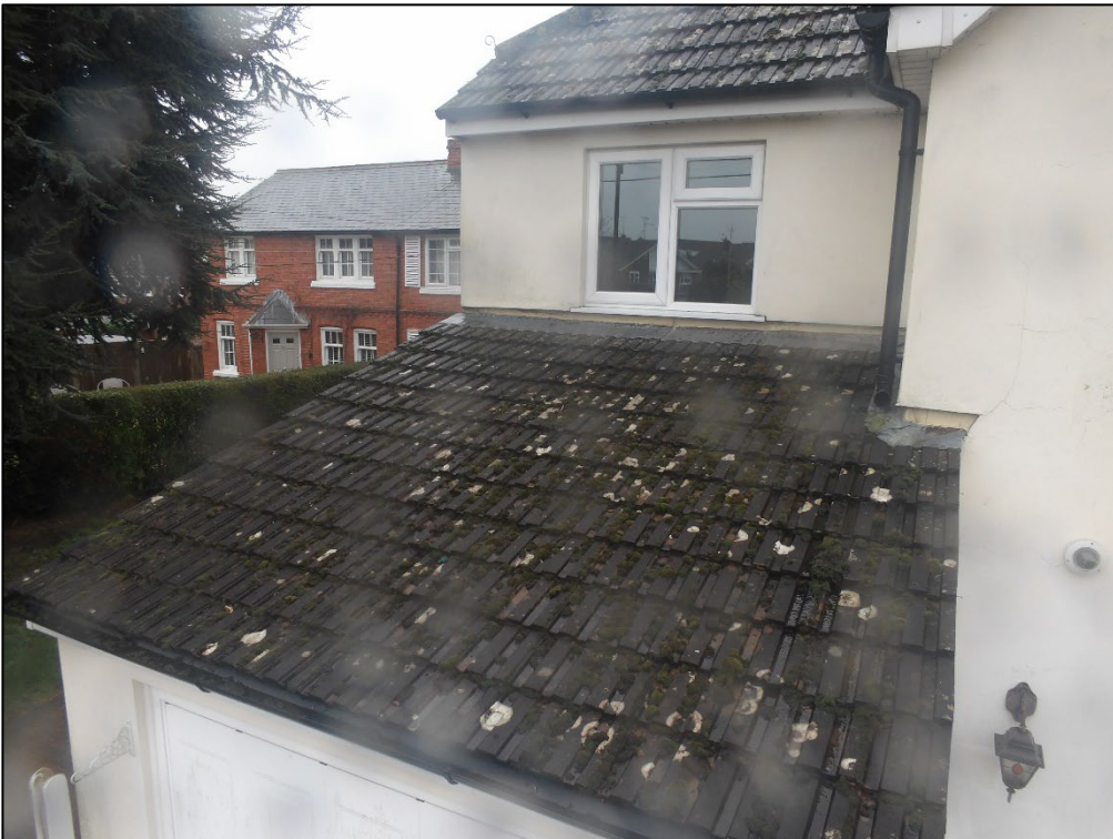
Figure 10. Garage roof. 52 Oatlands Road, Shinfield. 08.02.24
