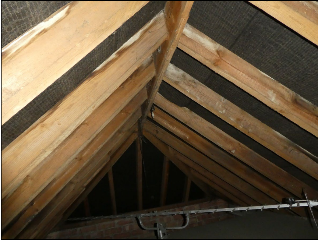
Figure 12. Example bitumen lining to roof tiles. 52 Oatlands Road, Shinfield. 08.02.24
