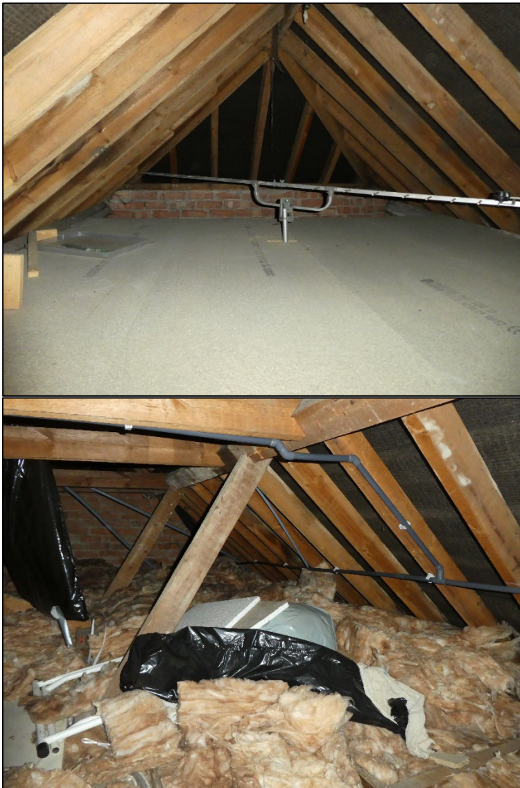
Figure 11. Example loft space. 52 Oatlands Road, Shinfield. 08.02.24
