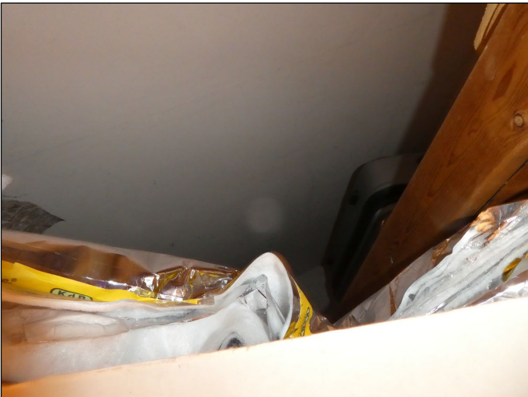
Figure 11. Example remaining garage roof space. 52 Oatlands Road, Shinfield. 08.02.24
