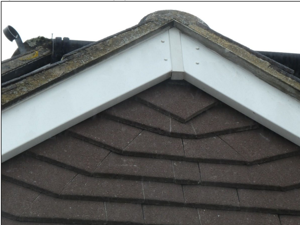
Figure 6. Example sealed hanging tiles. 52 Oatlands Road, Shinfield. 08.02.24
