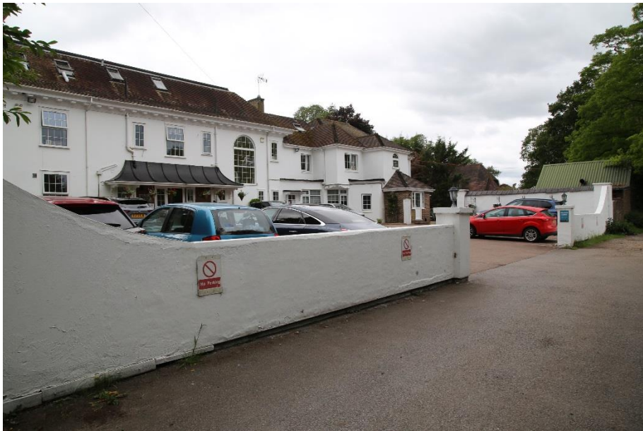
Plate 1 – Warren Lodge Care Centre is a large building with various extensions, it is located towards the end of Warren Lane.
