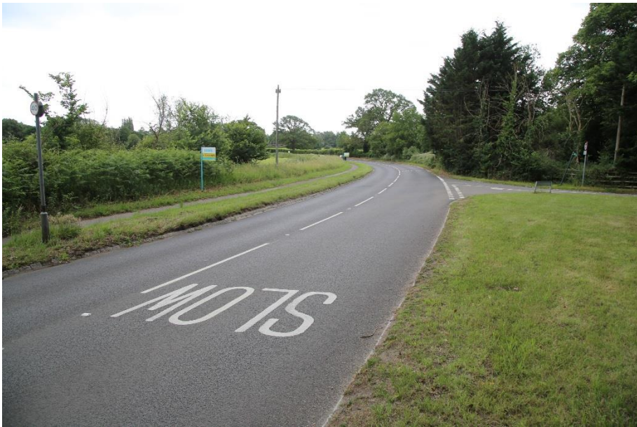
Plate 8 – SLOW warning lettering painted onto the B3106 beyond the Site to advise motorists of their approach to Finchampstead and a 30mph zone.
