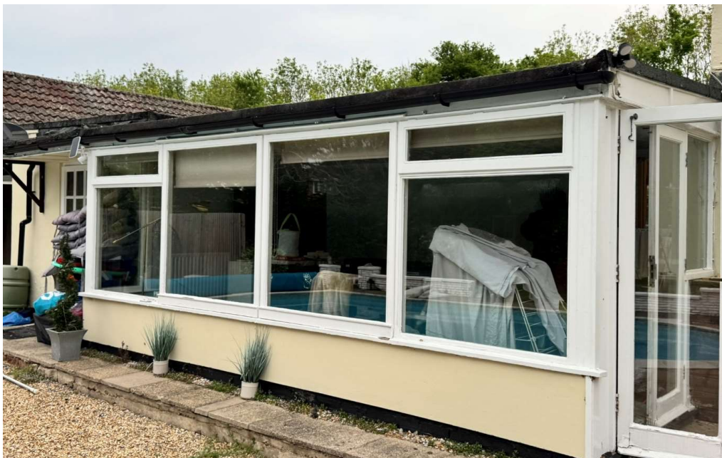
Pic. 1 – Existing Single Storey Wing & sun room
