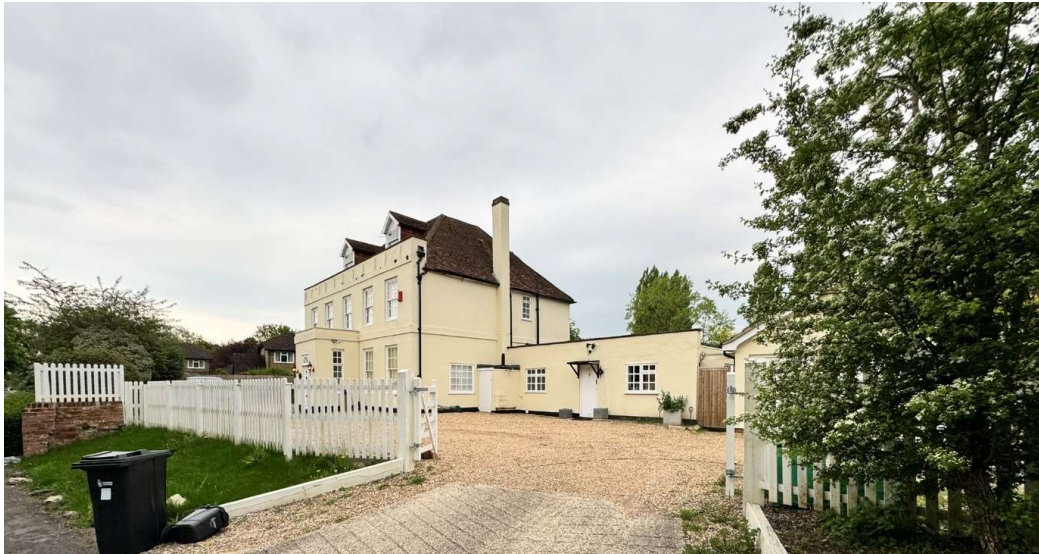
Pic. 4 – Existing House, Wing & Garage (Front Elevation from Road)
