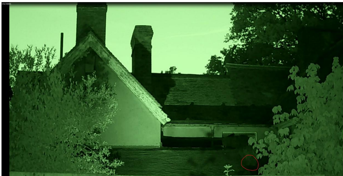
Image 3. Image of a screenshot showing a Common Pipistrelle emerging from Building B9
