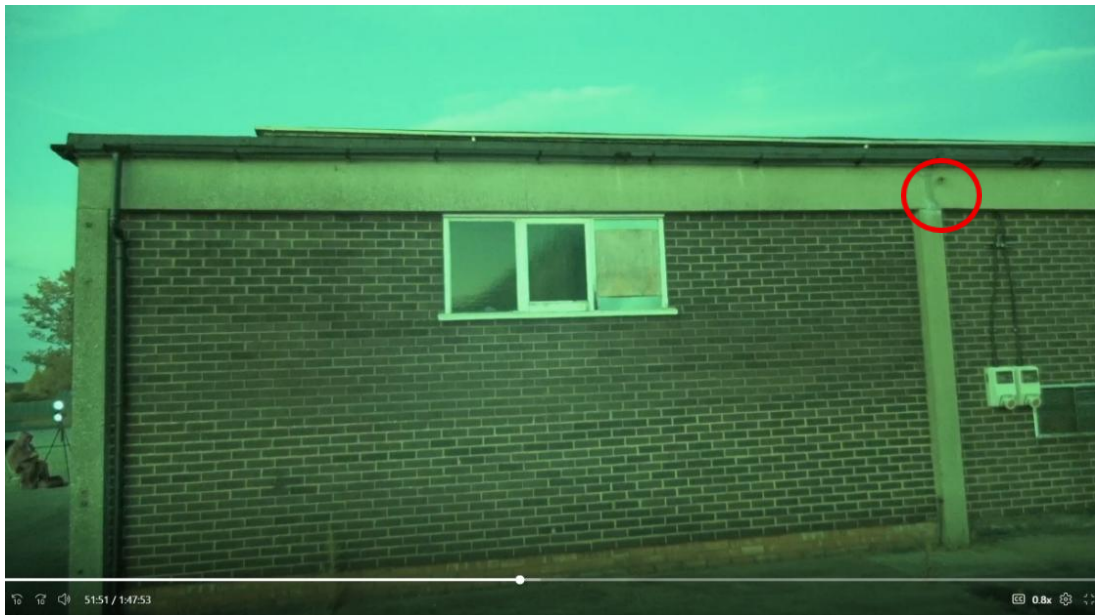
Image 2. Image of a screenshot showing a Common Pipistrelle emerging from Building B4
