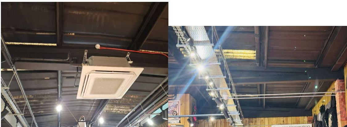
Below, Fig 3a +3b showing internal view of existing roof.
