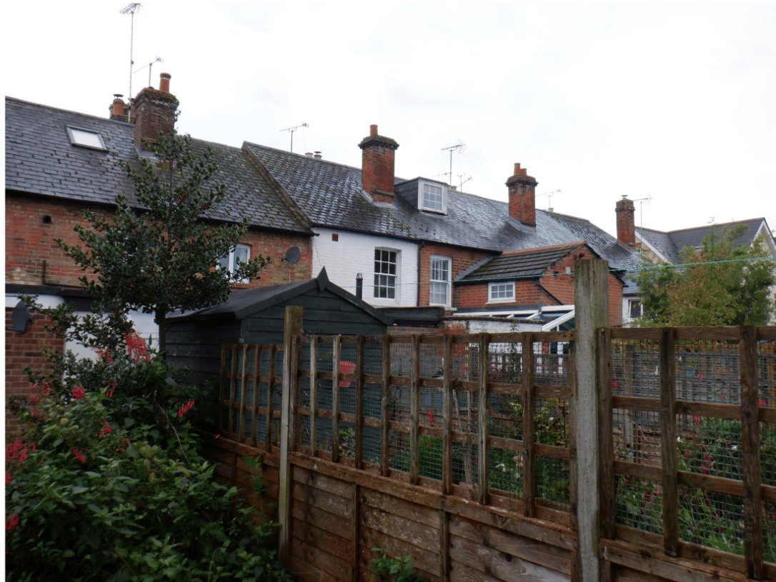
Rear view showing first floor rear extension to another property in the terrace
