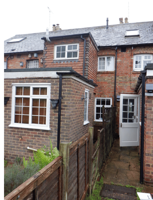
Rear view showing neighbour's existing first floor bathroom
