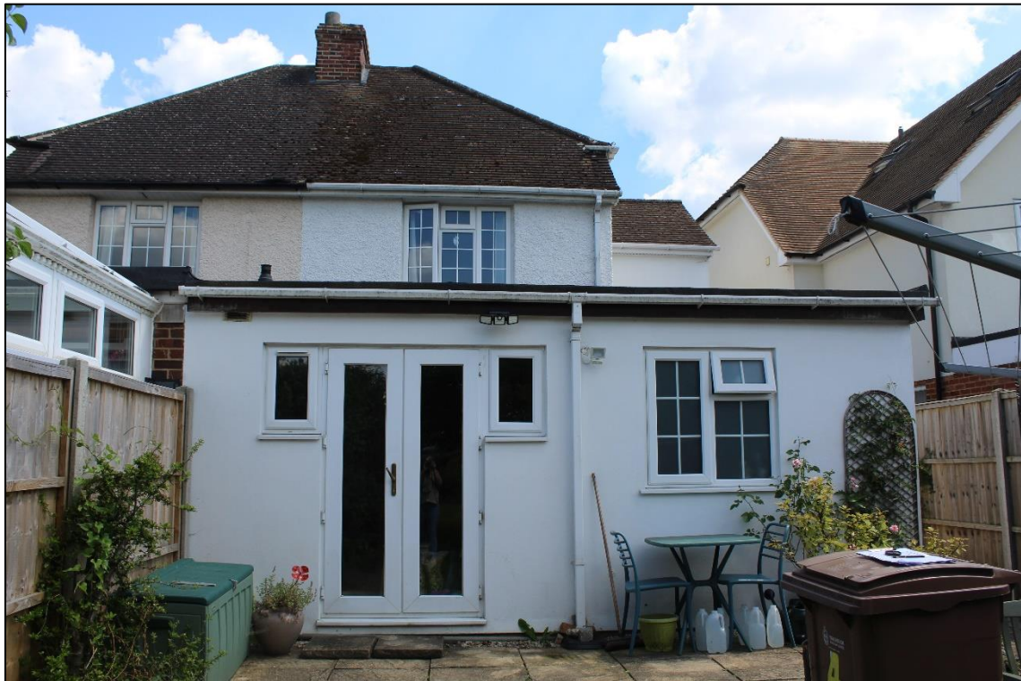
Photograph 3 – Rear elevation showing the single-storey extension completed in circa 1998
