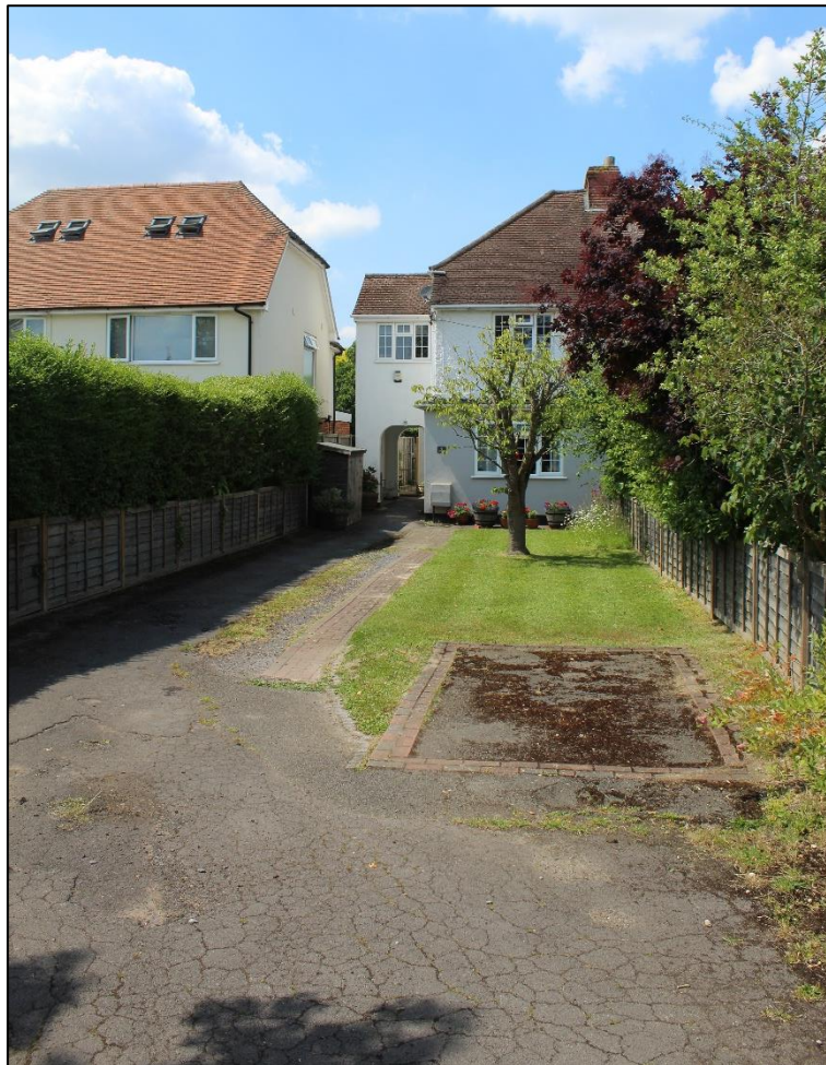
Photograph 1 – Front elevation as viewed from the driveway
